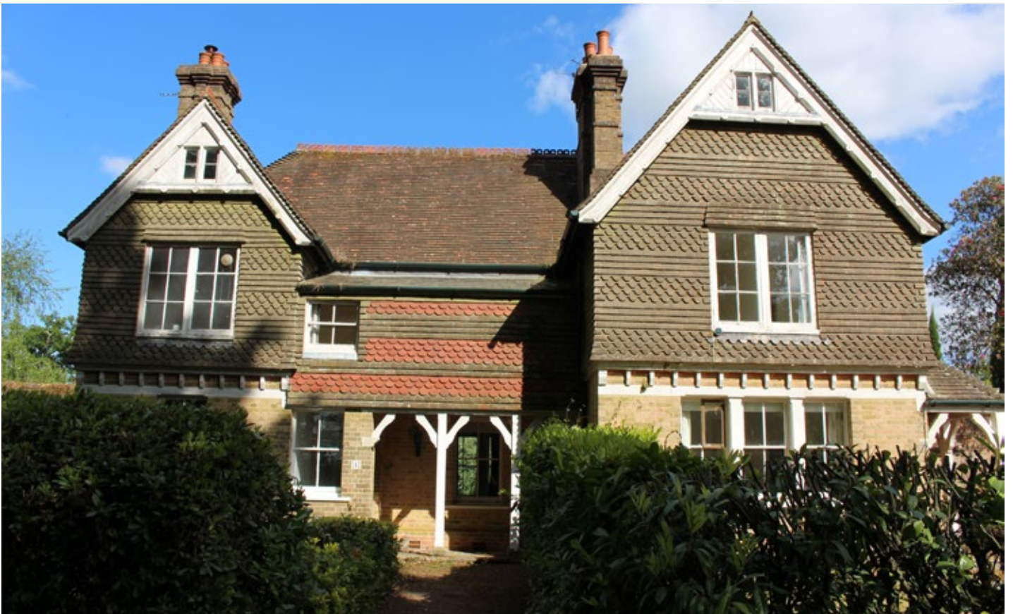
The western elevation of the cottages with different style and materials suggesting later addition. Noted in the history approval granted in 1901 for a Bothy, perhaps a rebuild or major addition to building shown on 1874 OS map.
