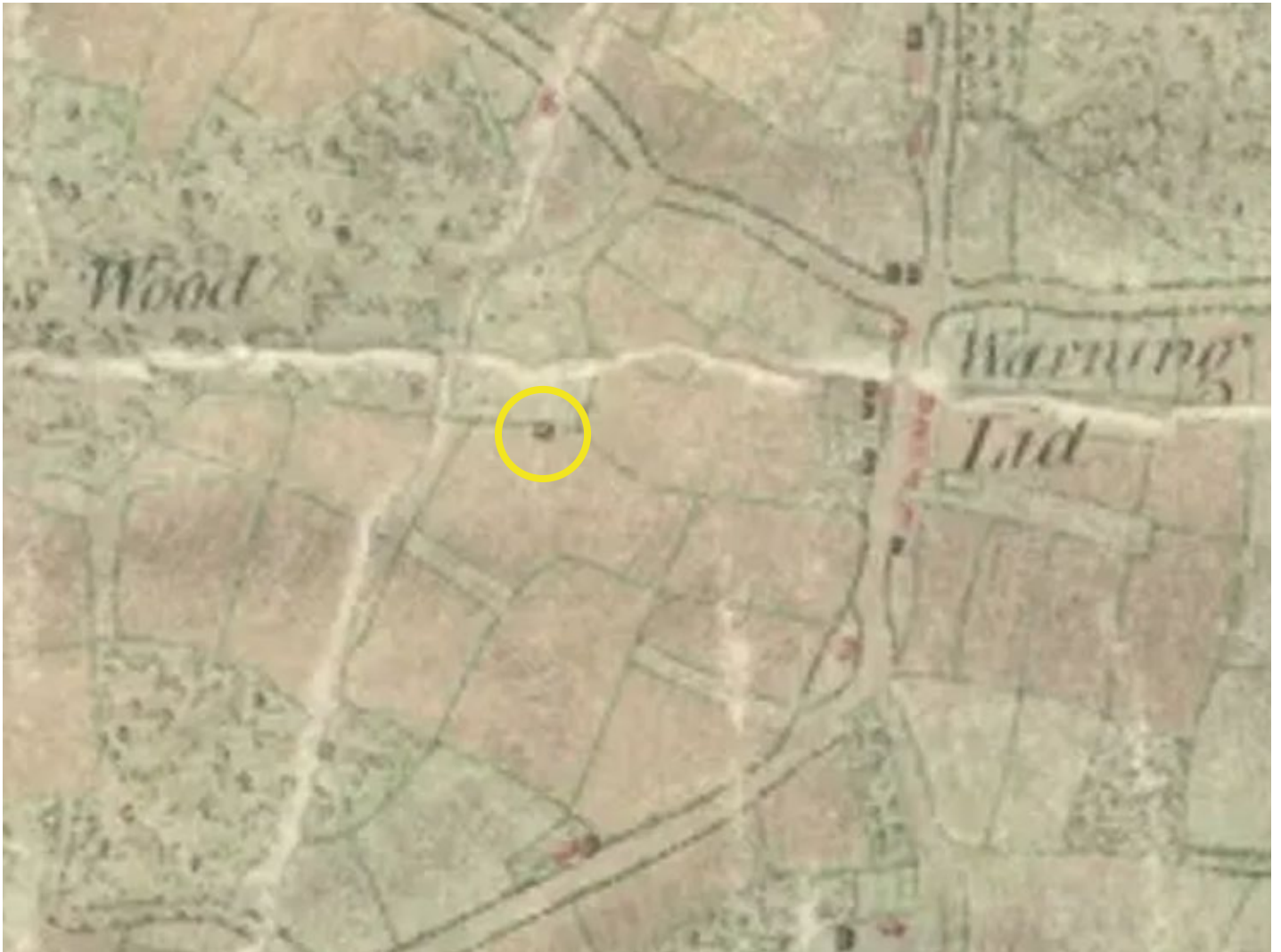
Extract from the survey of 1797 of the area around Warninglid which shows a building (yellow) to the west of the village on the site of the current Lydhurst
