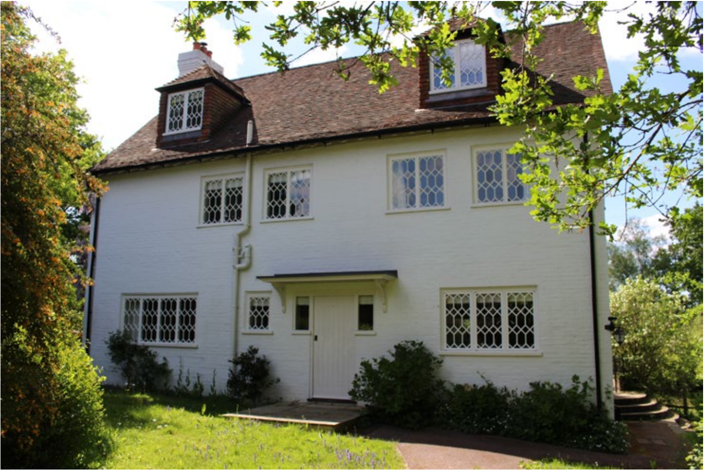
House to west of estate yard. Detached house to the west of the estate yard shown on the 1909 OS map.
