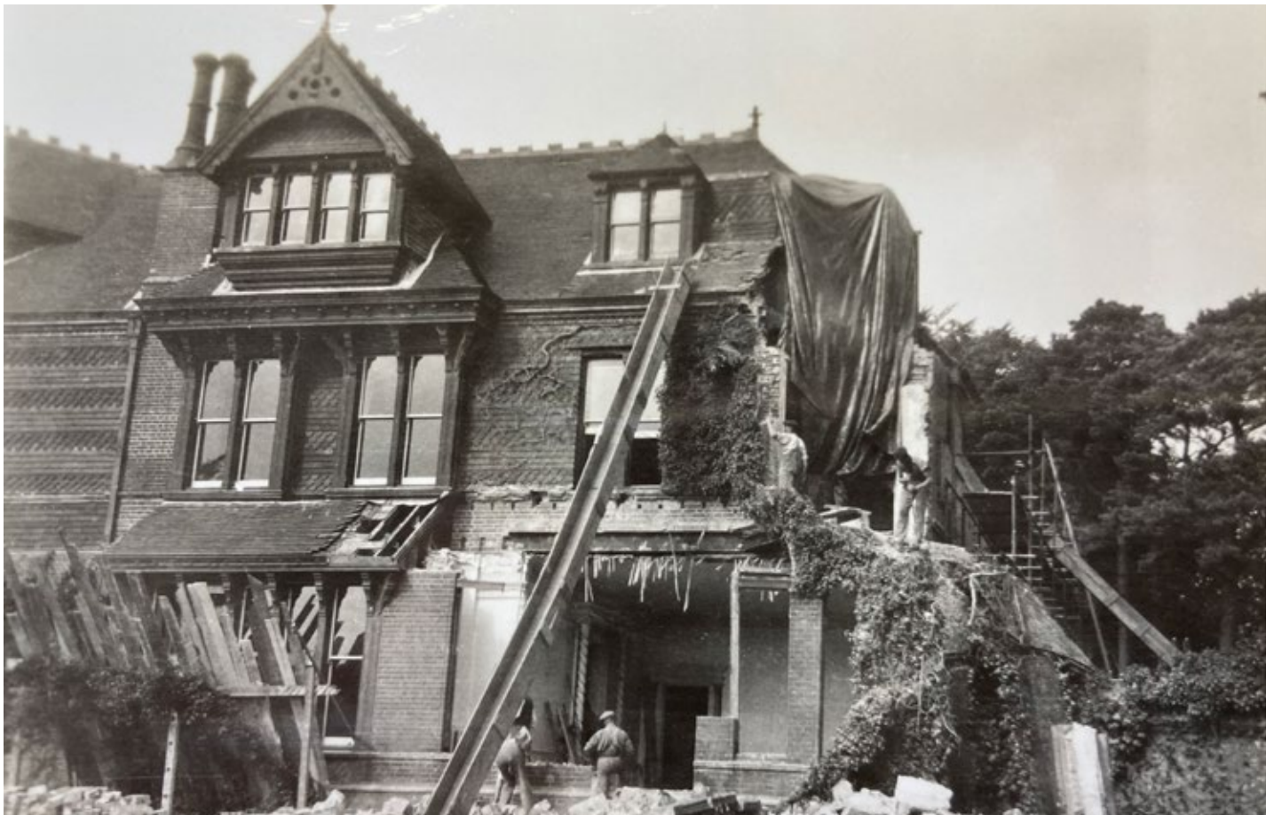
House being demolished (West Sussex Record Office ref: AMA818/3/2/6) (image 14 25 18)
