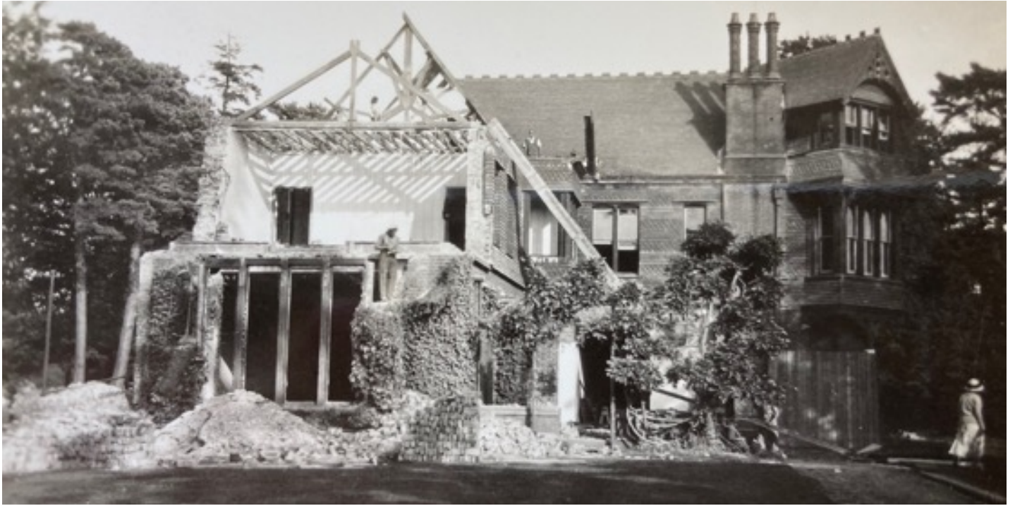
House being demolished (West Sussex Record Office ref: AMA818/3/2/6) (image 14 26 27)
