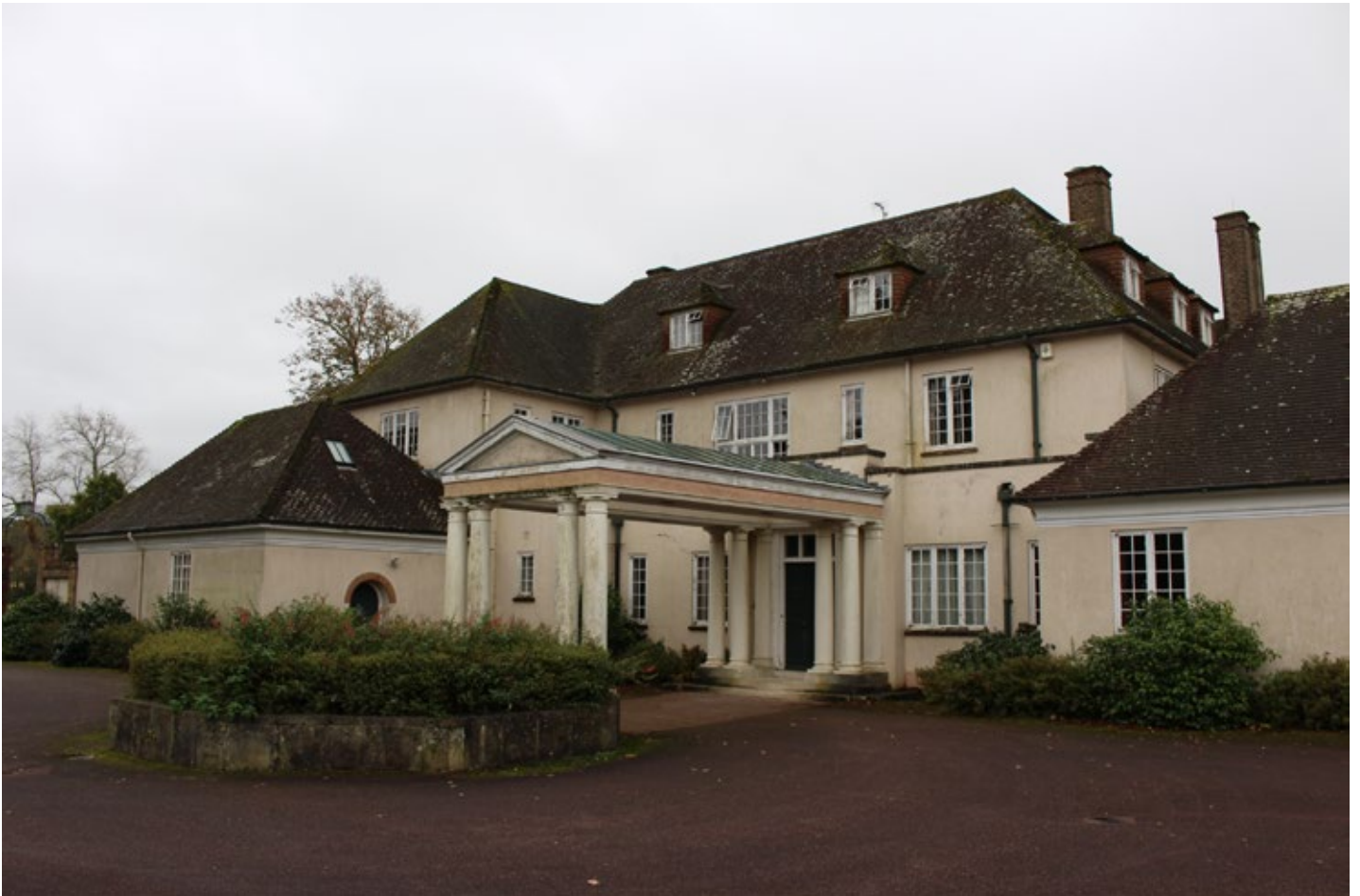
The north entrance elevation of the house showing later additions
