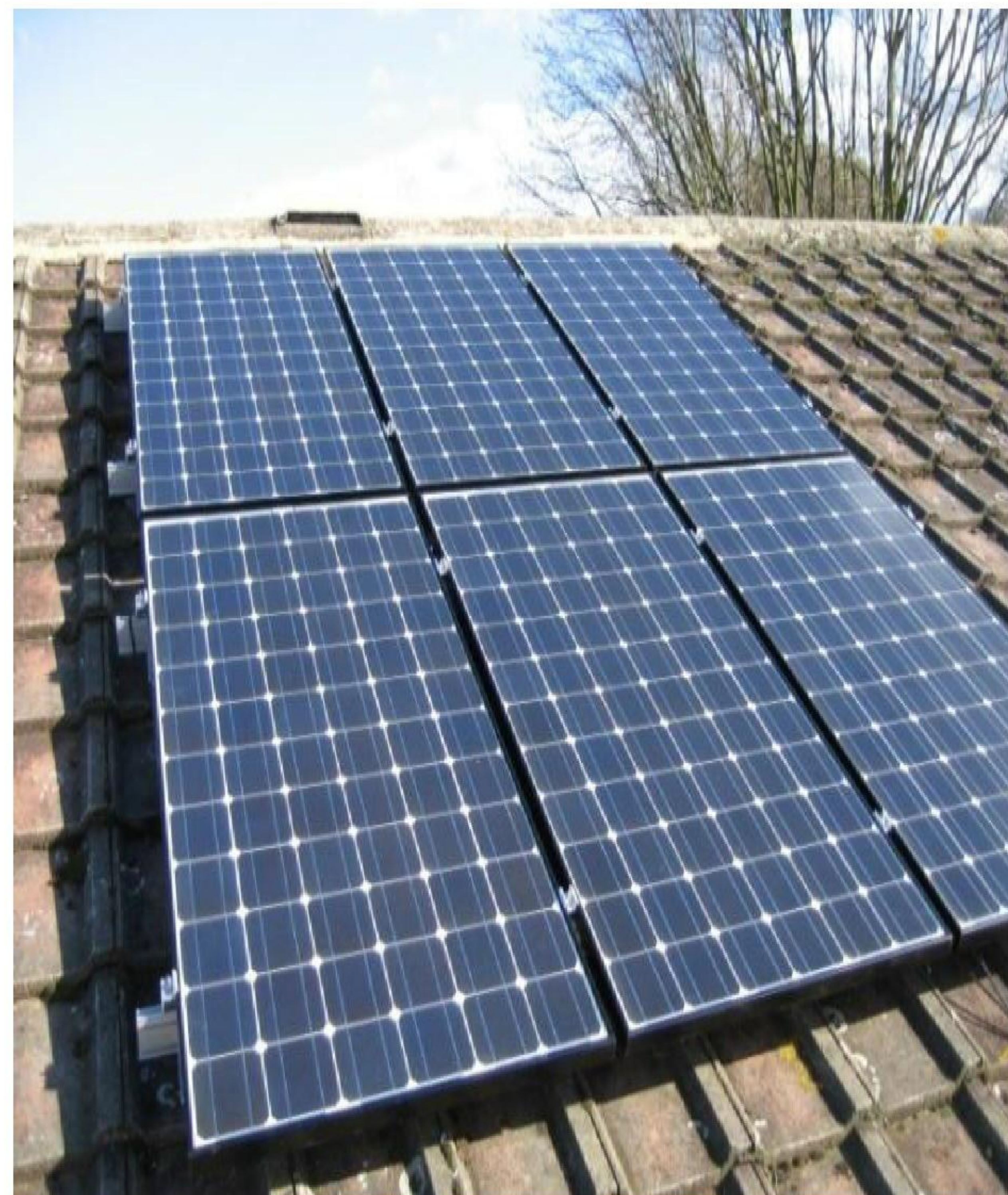
Figure 6 - Photovoltaic array on a pitched roof
