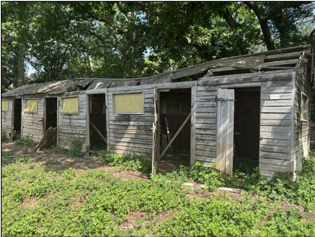
Figure 2 – Image of Stable Block
