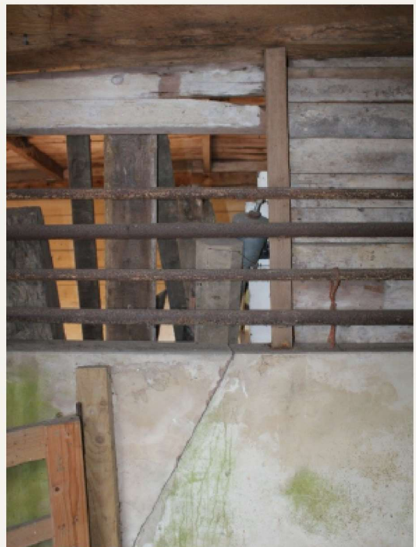
Image of the concrete rendered half height wall
