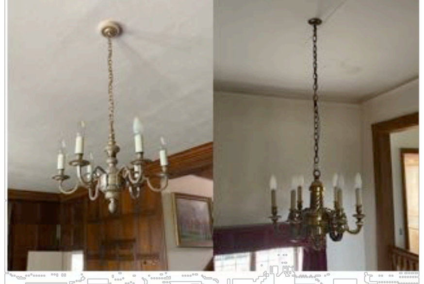
Chandeliers Chandeliers to be rewired and refurbished if required.
