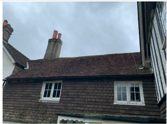
Front roof slope and chimney stack of the original roof.
