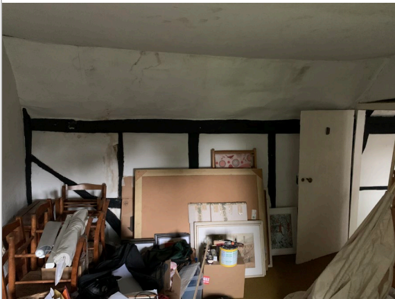
View of first floor bedroom looking towards location of proposed roof lights
