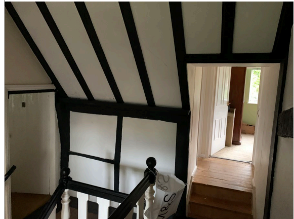
View of first floor stair landing
