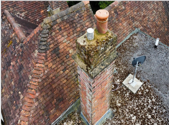
Original pitched roof to flat roof junction
