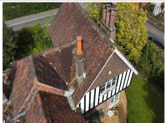
Pitched roof to original house and 19th Century extension
