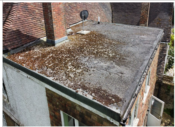
Flat roof to 1970 extension
