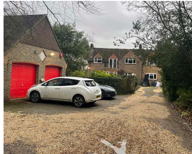
View of existing garage and house in the background
