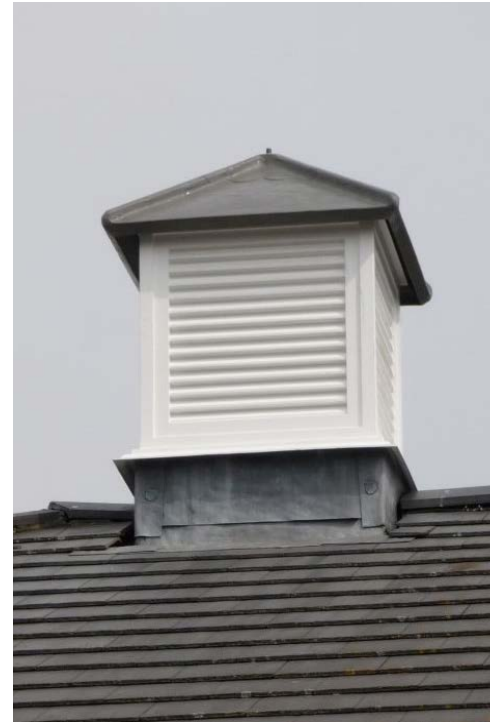
Roof Turret / Dovecote tower
