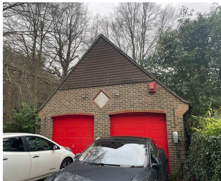
Original Garage informing the design of the extension
