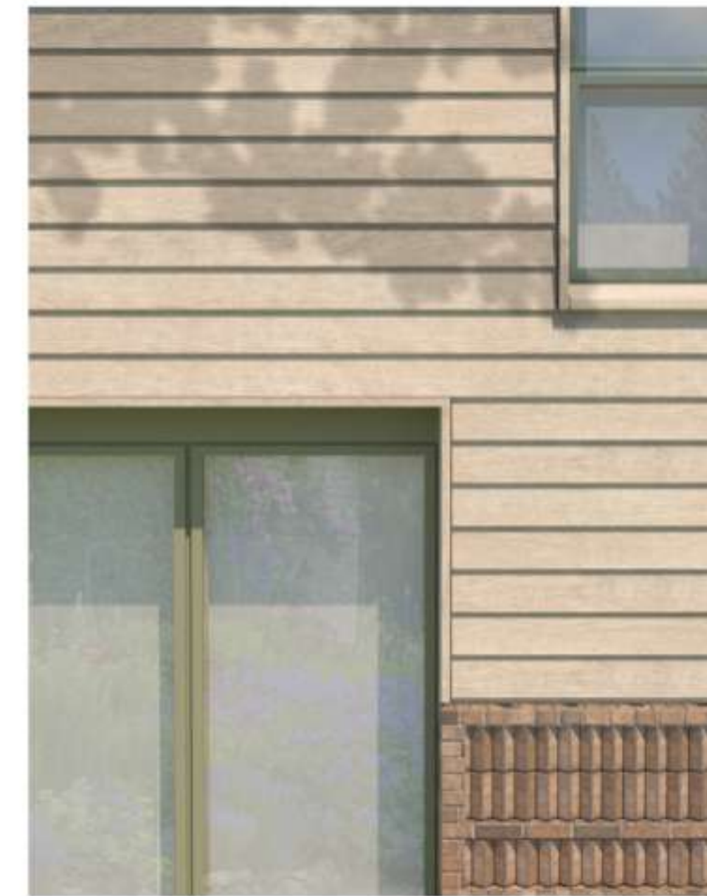
Window and door detail, brick plinth and timber cladding.
