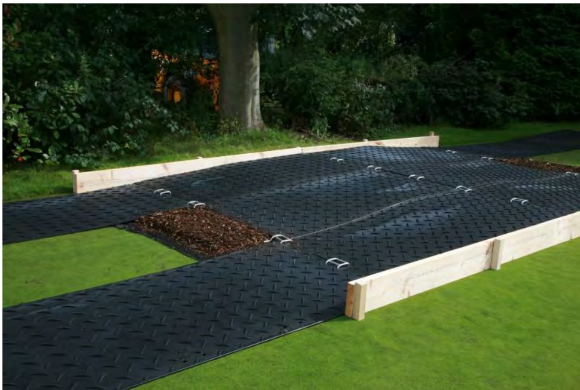
Figure 5 - Example of suitable temporary ground protection installation for pedestrian traffic and small plant
