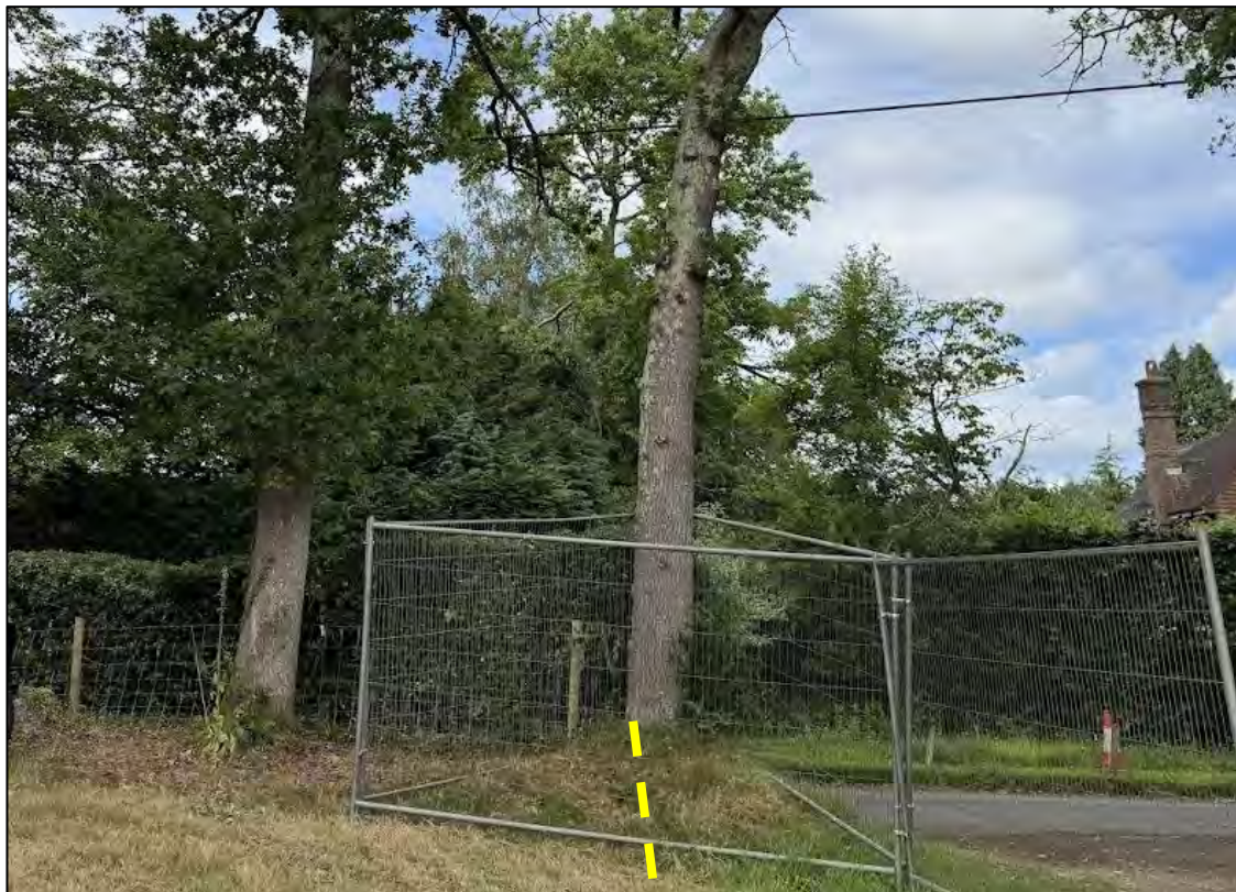
Figure 1 – Yellow dashed line indicating line of manual excavation required to widen access.
