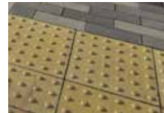
Blister tactile paving in buff
