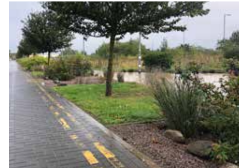
Wetland planting with crushed aggregate and boulders along roadside. (Cambridge North Station Source: James Dee / AECOM 2023)
