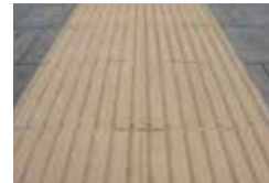
Corduroy Paving in buff
