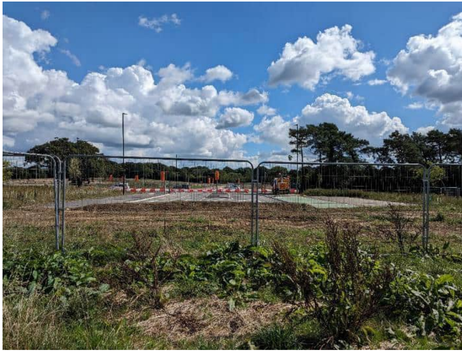
Plate 17. The existing Eastern Bridge and Link Road at the proposed tie-in location to the proposed Central Section, looking east. Photograph taken 12/09/2024
