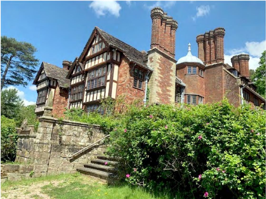
Plate 9: Garden wall and Steps to terrace viewed from south
