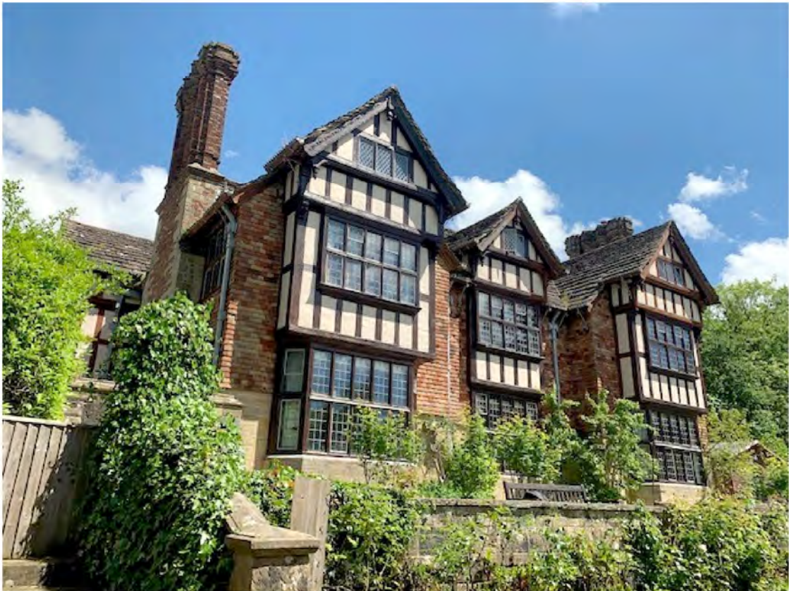
Plate 8: Southwest elevation viewed from level below terrace
