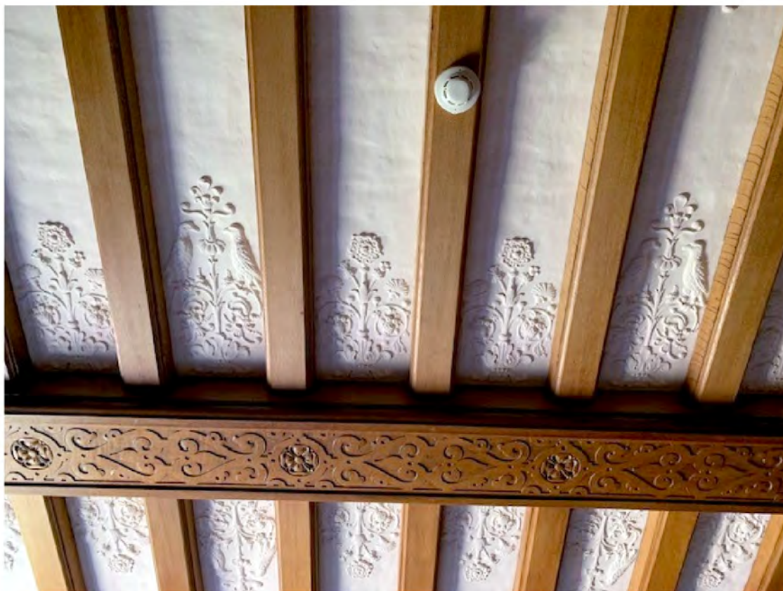
Plate 23: Study detail of ceiling
