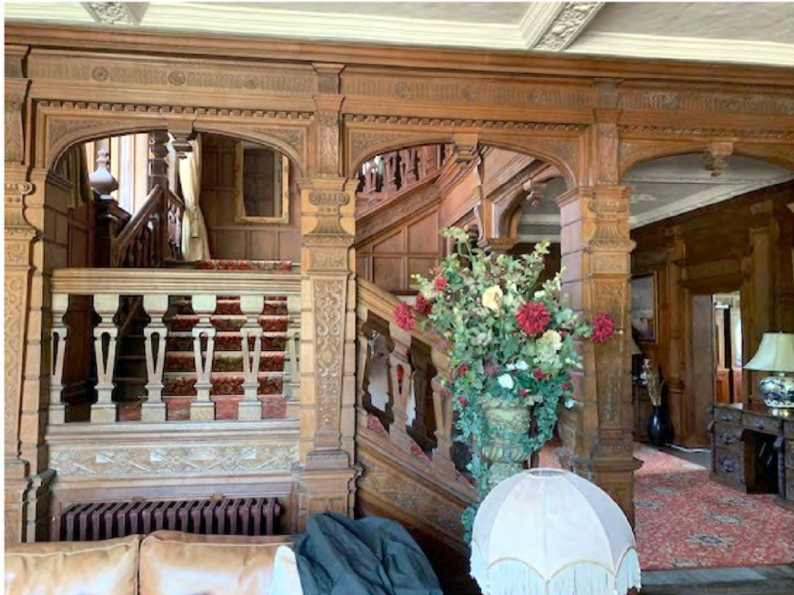
Plate 15: Entrance Hall looking southeast towards staircase
