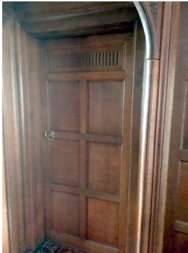
Plate 33: Door, ironmongery and panelling to first floor
