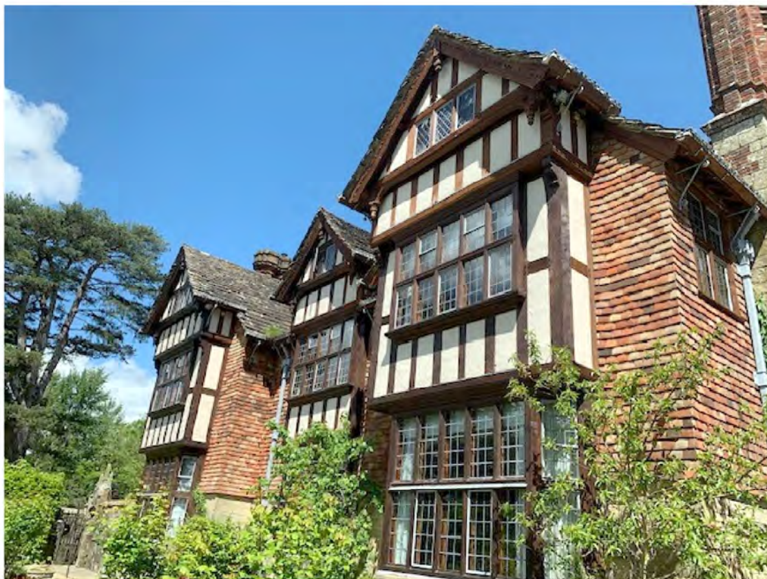
Plate 11: Southwest elevation from terrace
