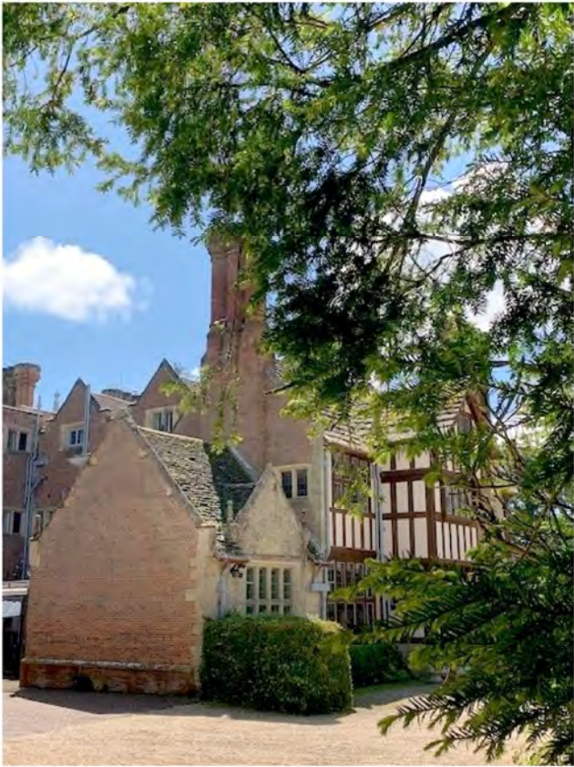
Plate 3: North corner of Chownes Mead viewed from north
