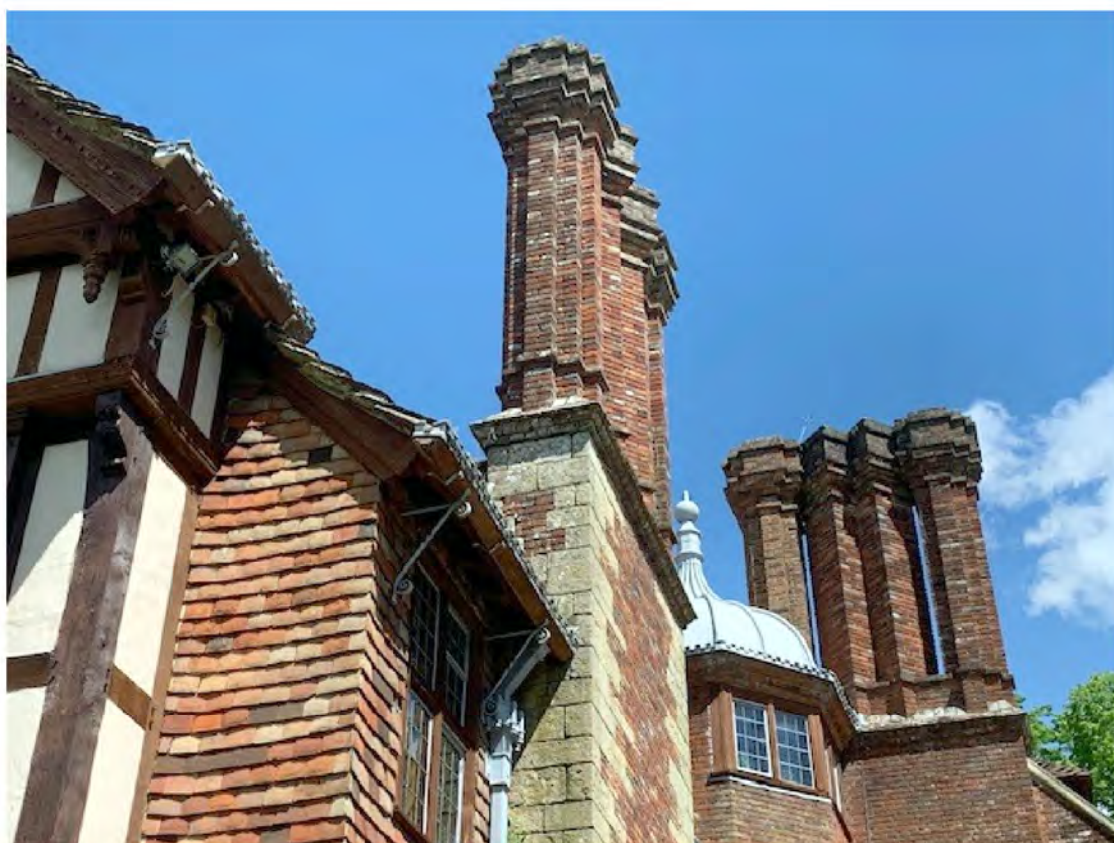
Plate 14: Southeast elevation - corbelled chimneys
