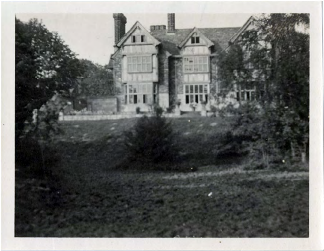
Plate 10: Archive Image sent of works to Gertrude Jekyll - southwest elevation
