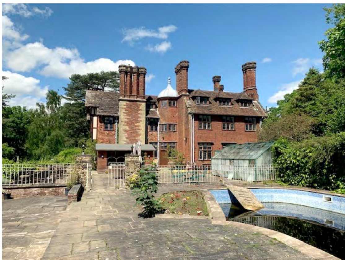
Plate 12: Southeast elevation beyond swimming pool
