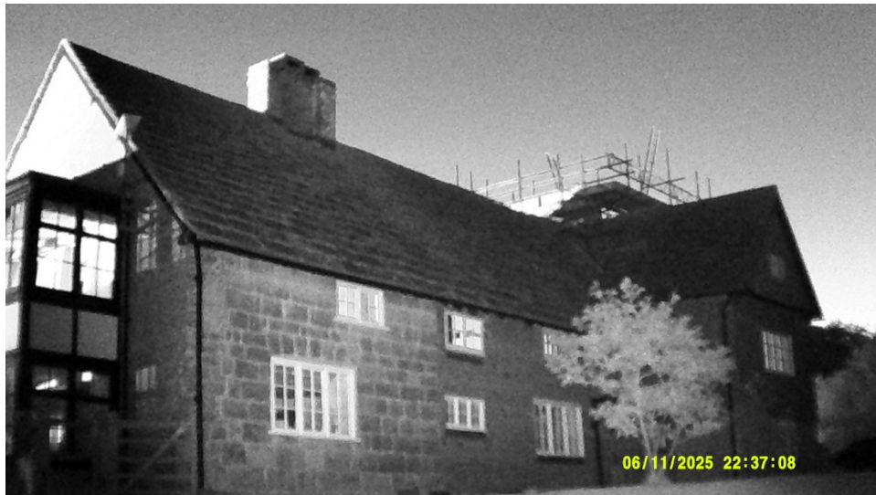
Image 7: IR View of Main House (south-eastern elevation)
