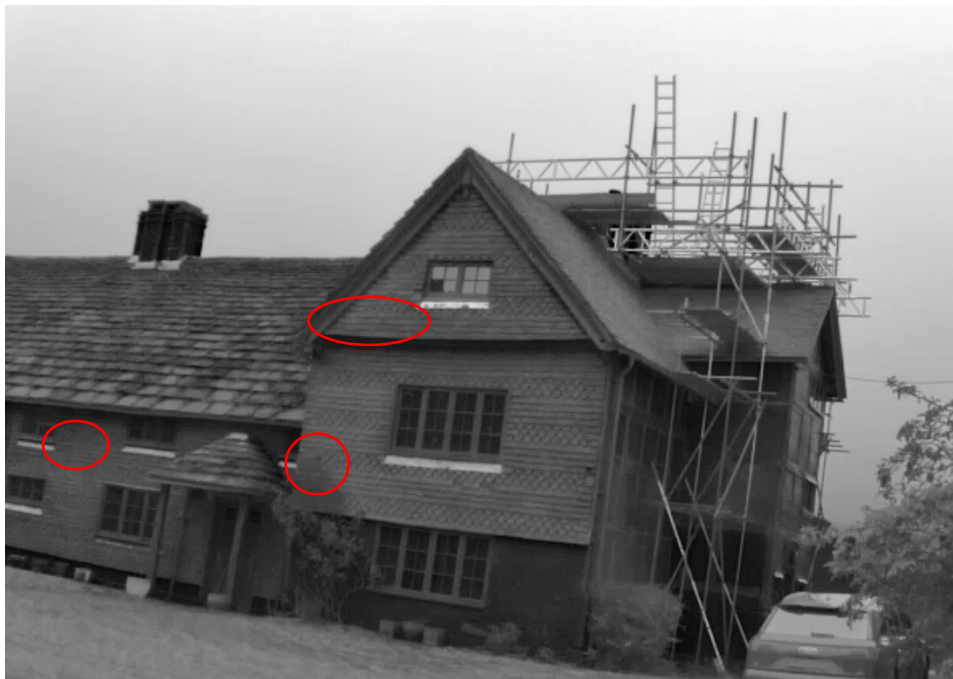
Image 4: Thermal imaging view of Main House (eastern elevation). Approximate roosting locations of common pipistrelles shown in red.
