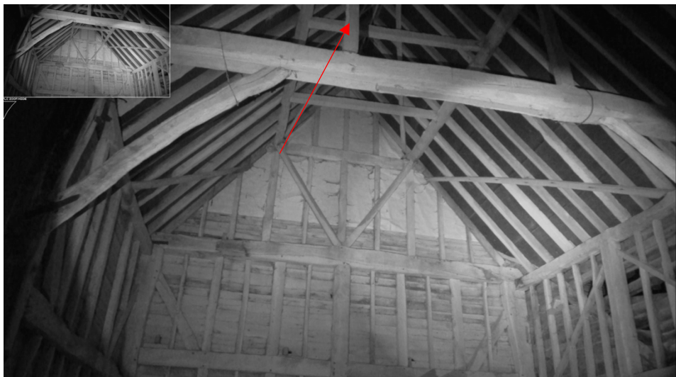
Image 2: Internal view of Barn. Approx. roosting location in ridge shown in red.
