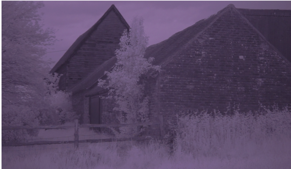
Image 3: IR View of Barn (Southern elevation)
