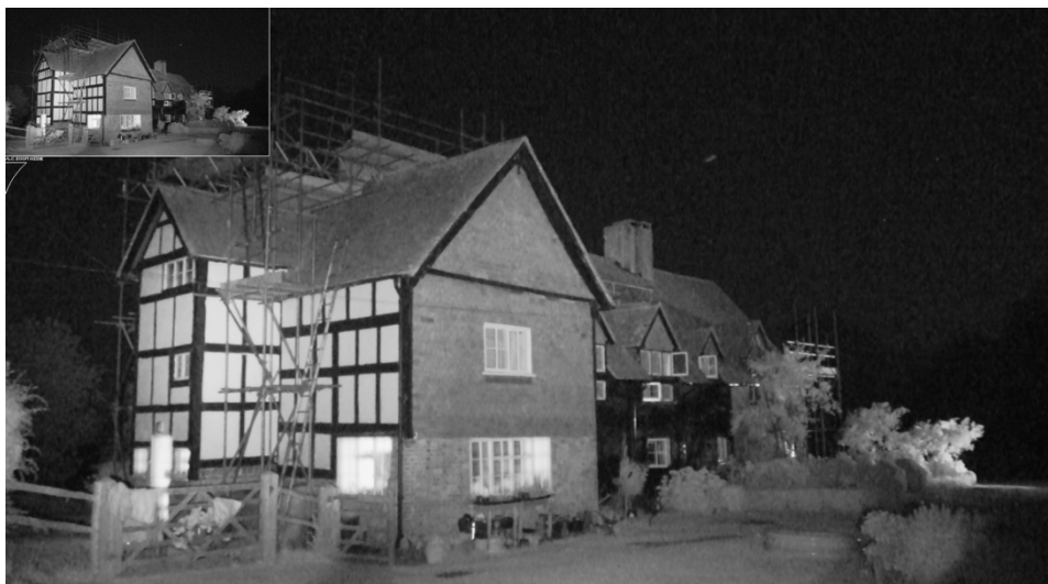
Image 6: IR View of Main House (Northern and western elevation)
