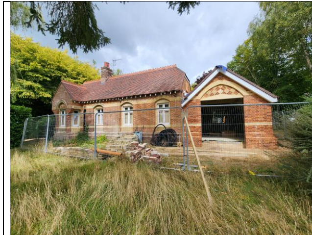
Photo 1: The residential dwelling (North Lodge).
