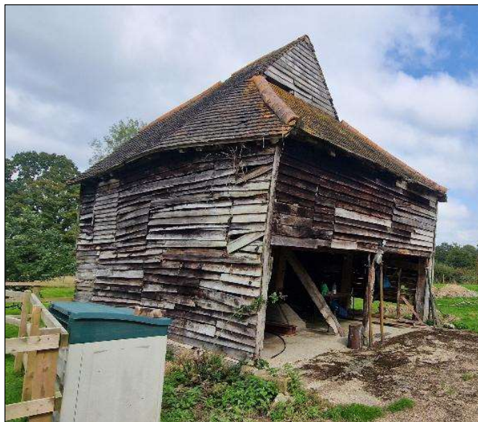
Image 1. Photo of The Granary building from he from the southwest.
