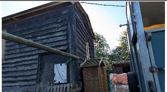
Photo 4: The north and west elevation of the barn.
