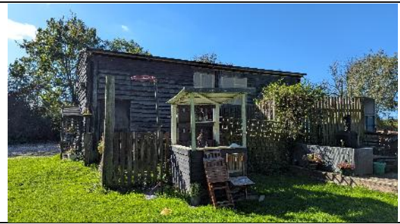
Photo 2: The north elevation of the barn.
