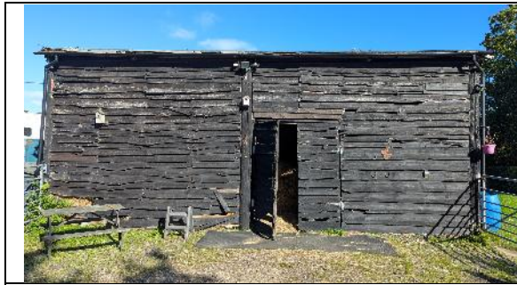
Photo 1: The southern (north) elevation of the barn.
