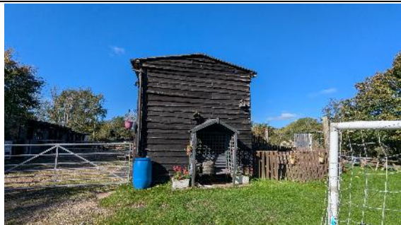
Photo 3: The north elevation of the barn.
