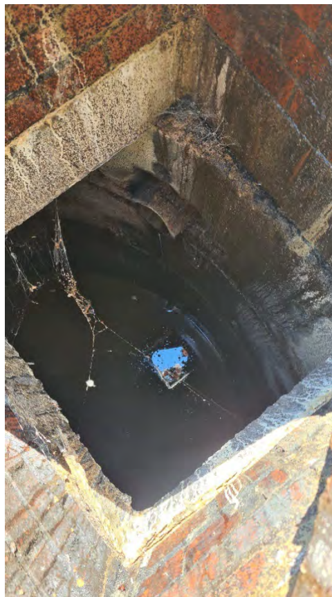
4. Looking into one of the soakaways that serves the site (June 2022)
