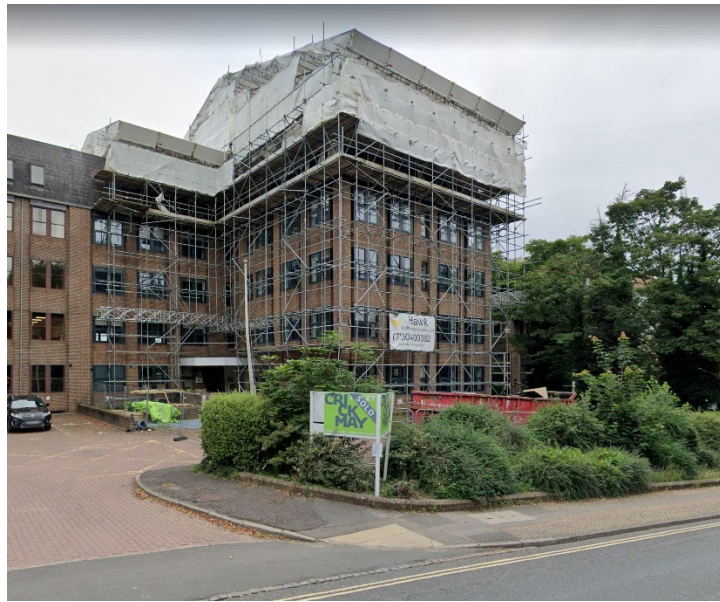
1. Front view of the site (Central House) – From Google maps (August 2021)
