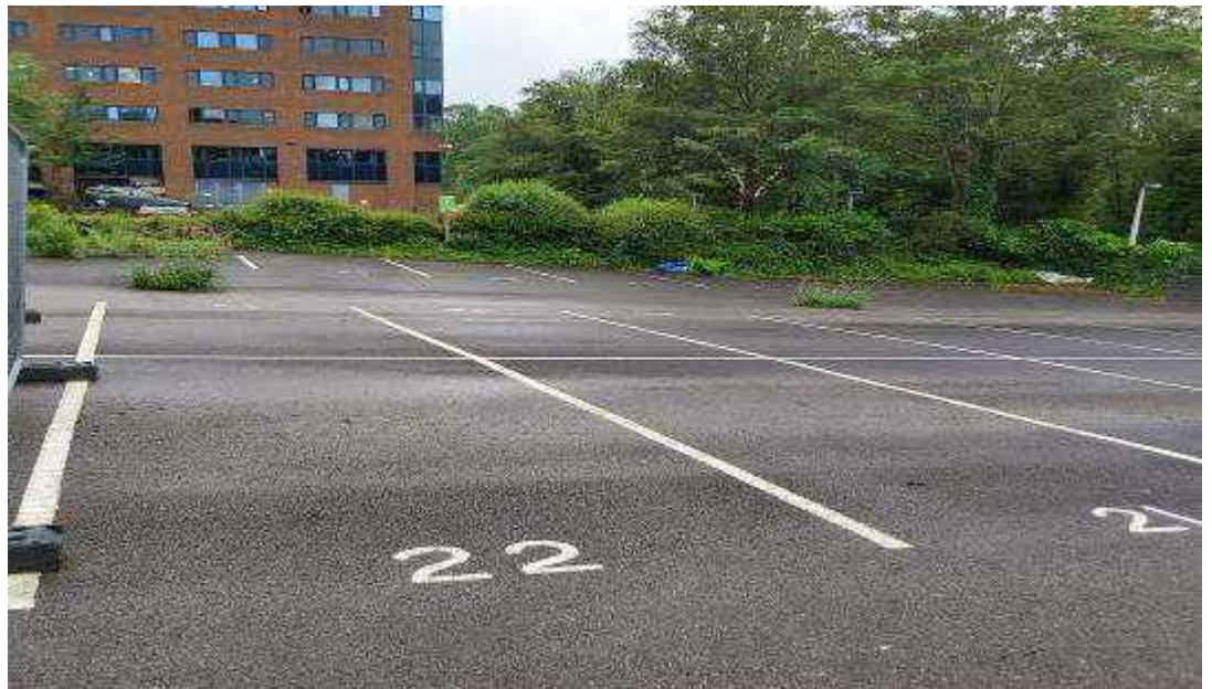
Car park and access road. (Proposed annex site)
