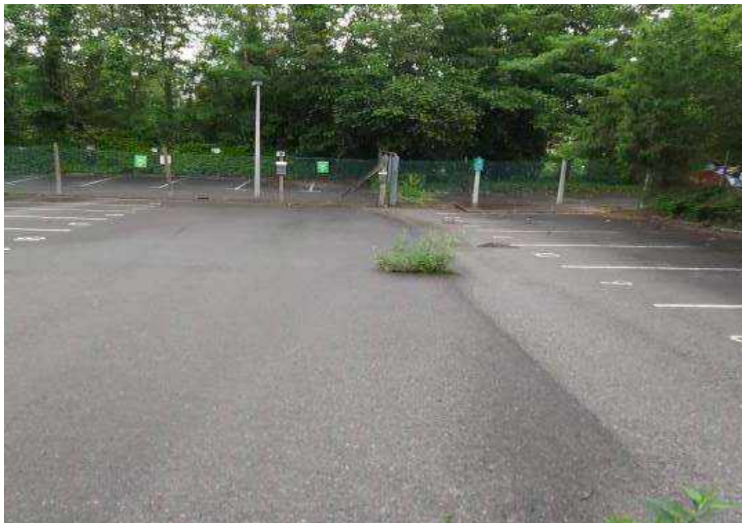
Car park. (Proposed annex site)
