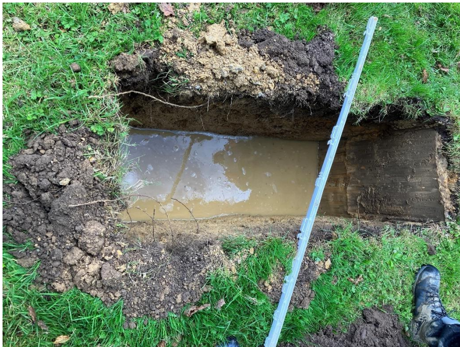
P4: Photograph showing TP08 during soakaway test.
