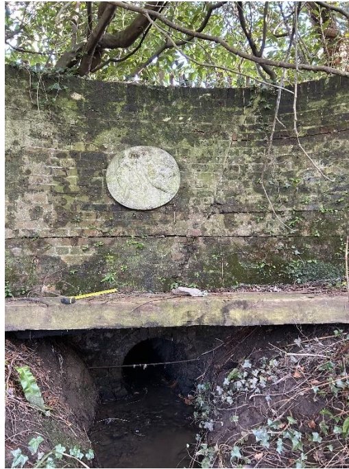
Figure 3-2: Culvert inlet
