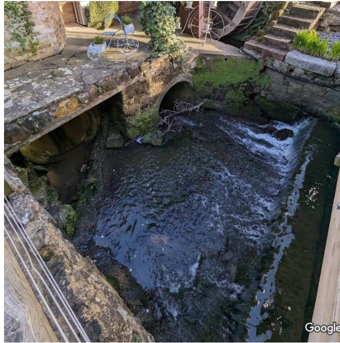
Figure 3-4: Dunning's Road culvert. Source: Google Maps
