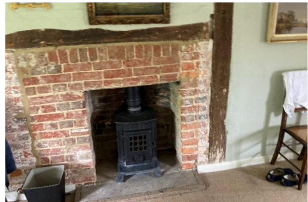
Figure 7 – Existing first floor fireplace
