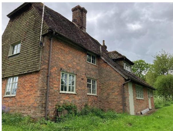
Figure 8 – Existing northwest corner
