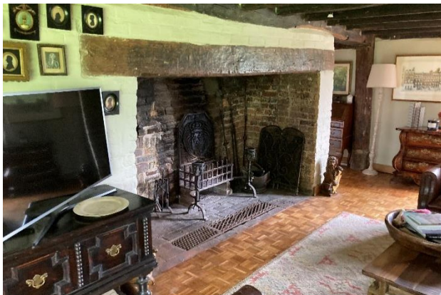
Figure 6 – Existing inglenook fireplace
