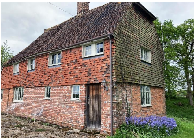
Figure 2 – Existing northeast corner
