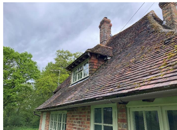
Figure 9 – Existing dormer window
