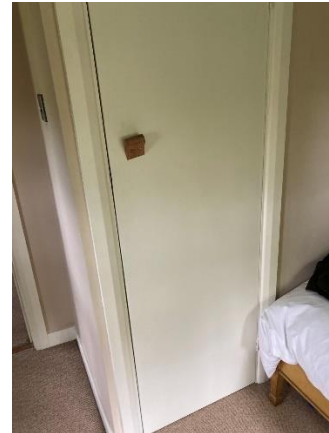
Figure 22 – Existing cupboard and internal wall to be removed
