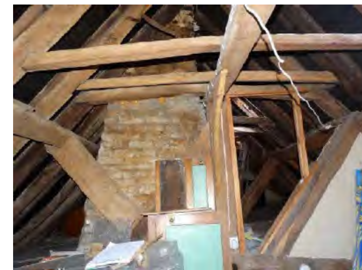
Attic, chimney stack in the background
