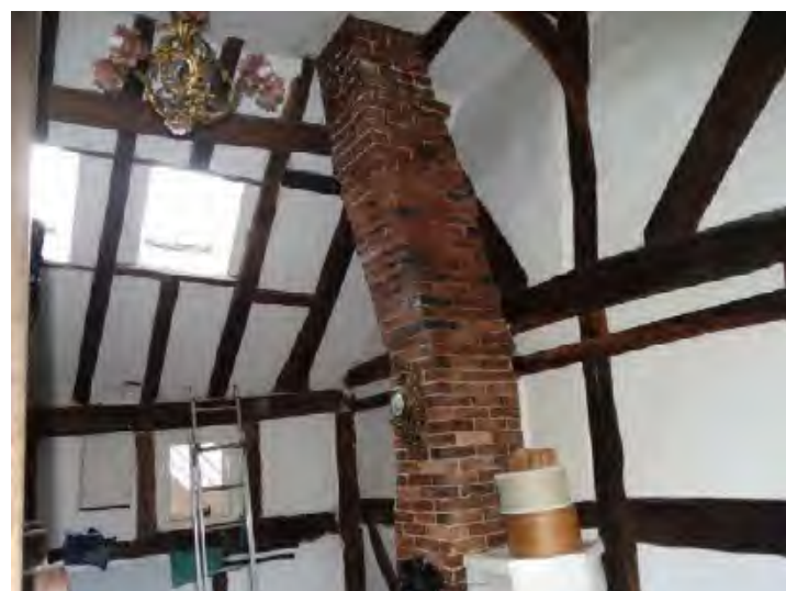
First floor bedroom, chimney stack
