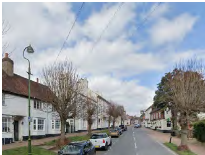
View looking North along High Street
