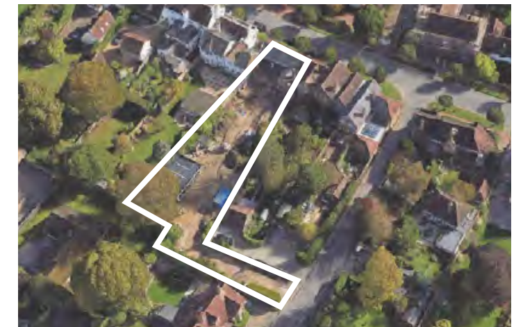
View looking East
