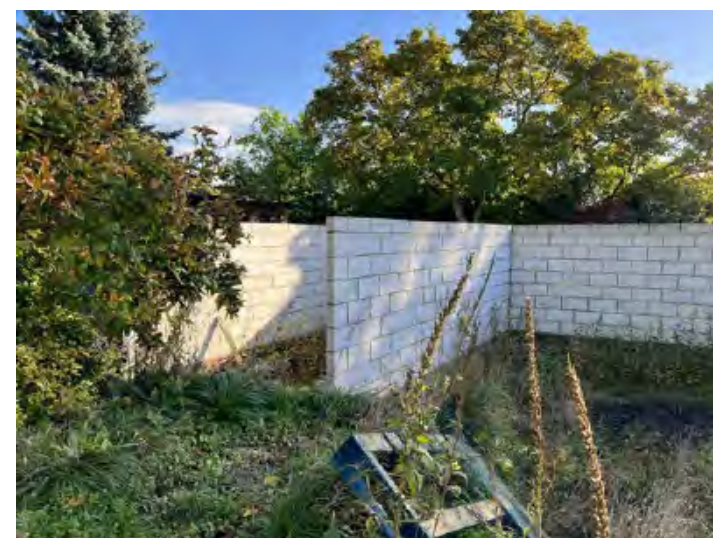
Garage walls constructed
