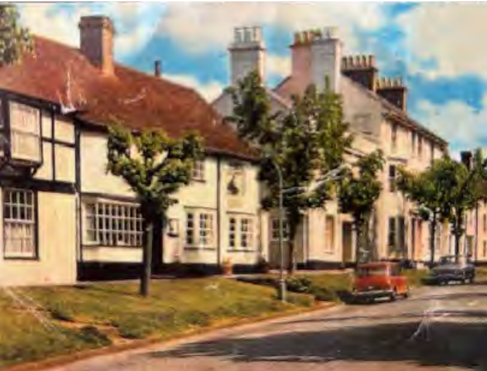
Historic photograph showing the original brickwork chimney
