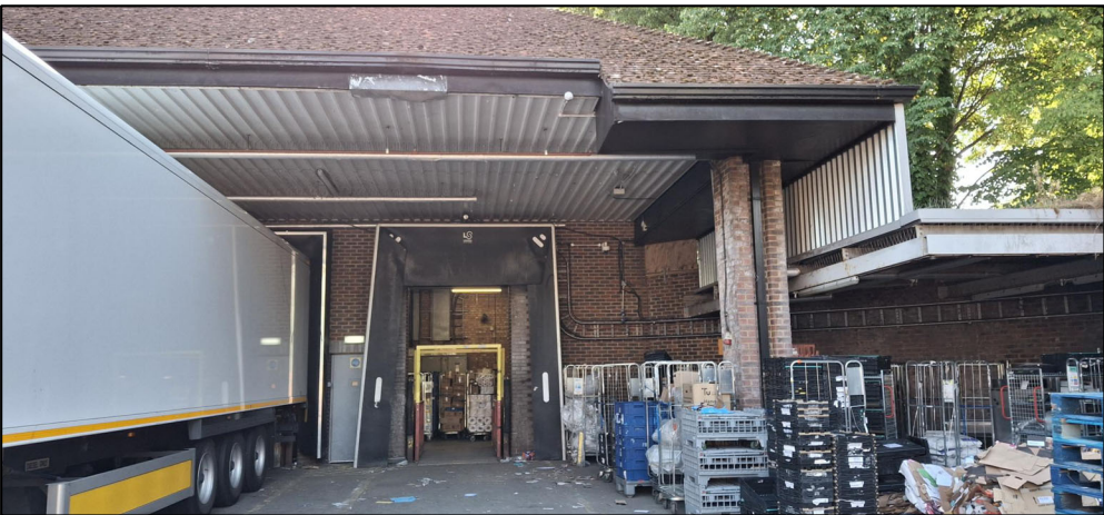
EXISTING UNLOADING BAY AREA PHOTOGRAPH
