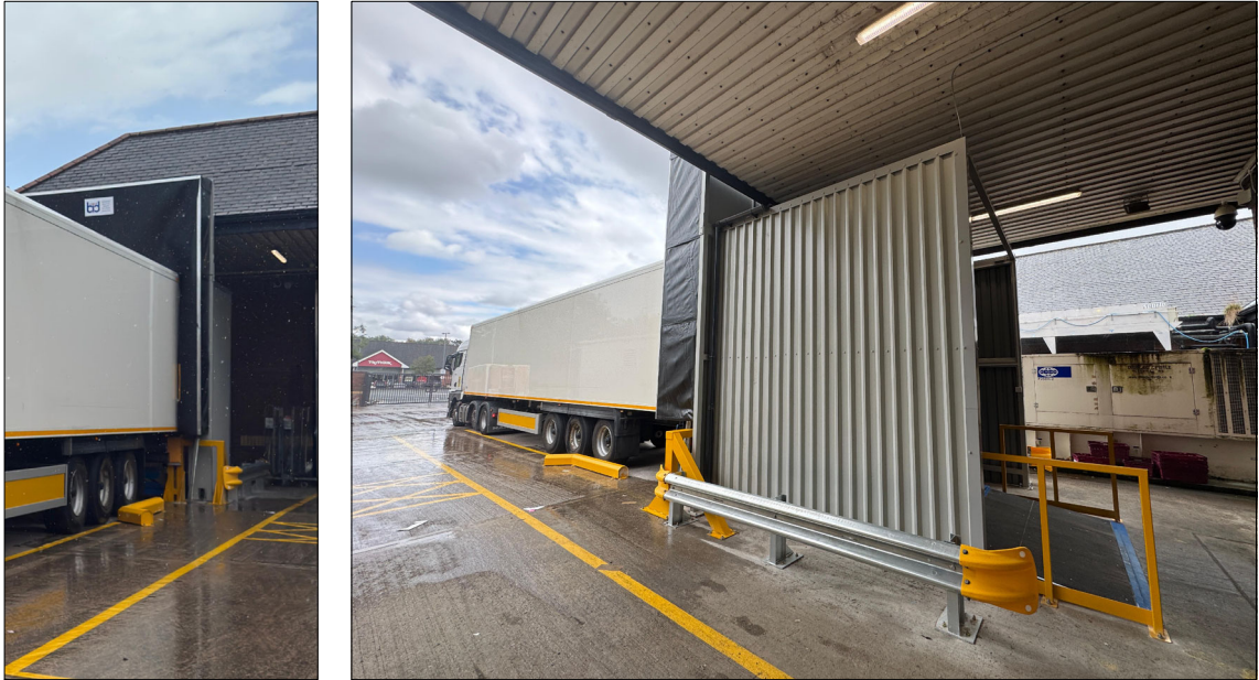
TYPICAL POD REFERENCE PHOTOGRAPHS
