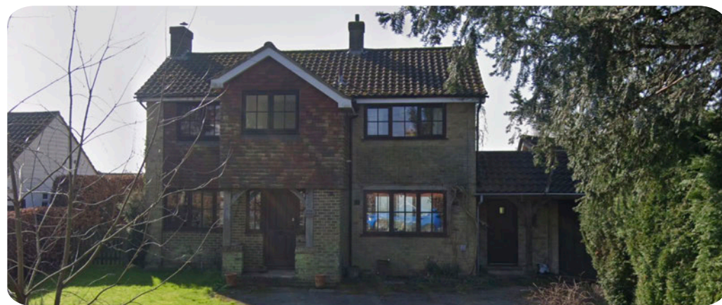
Front (North) Elevation (View from Cansiron Lane)
