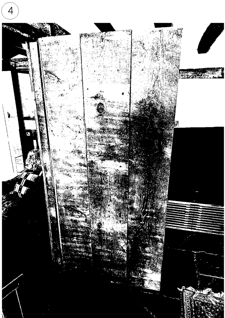
New timber plank door
