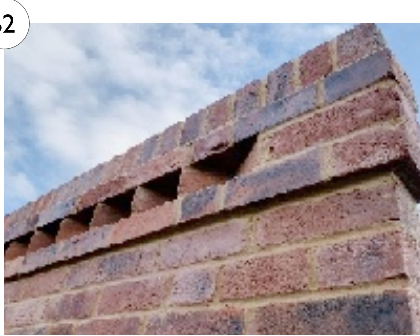
1.2M BRICK BOUNDARY WALL
