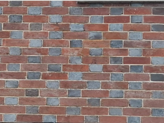
New brickwork to match existing as per above. Red brick with blue header
