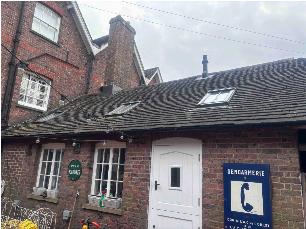
Photographs 2 & 3. 3no. conservation roof windows in ground floor rear (north) roof slope
