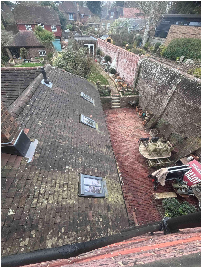
Photographs 2 & 3. 3no. conservation roof windows in ground floor rear (north) roof slope
