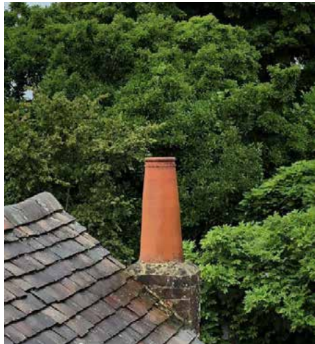
Original bake house chimney
