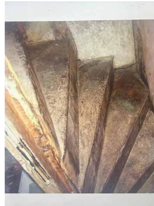
Staircase during demolition works
