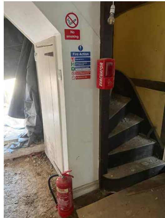
Staircase during demolition works
