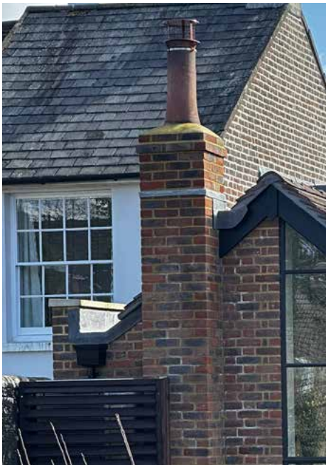
Recent photograph of parapet wall detail
