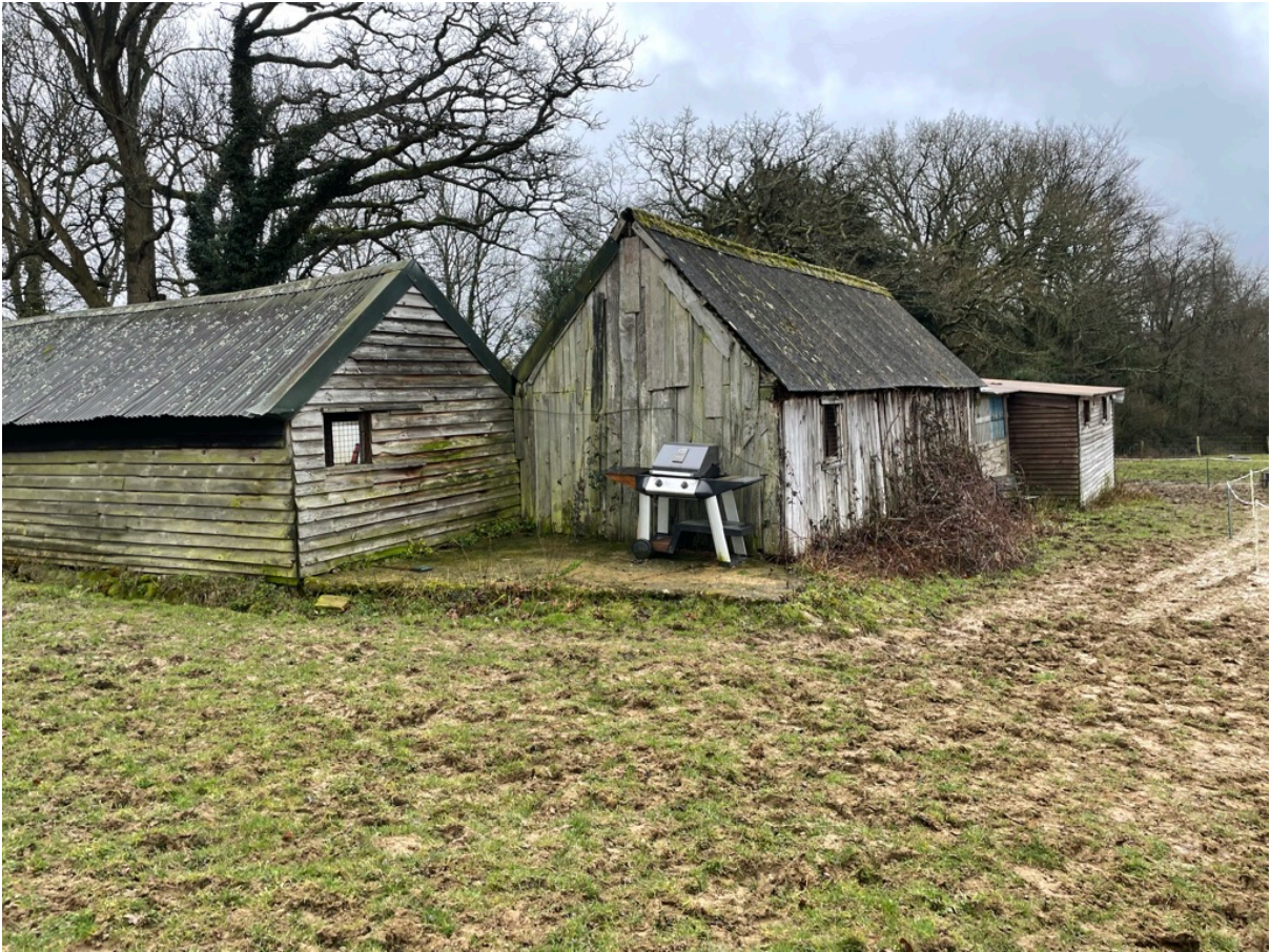
External View from the north-west
