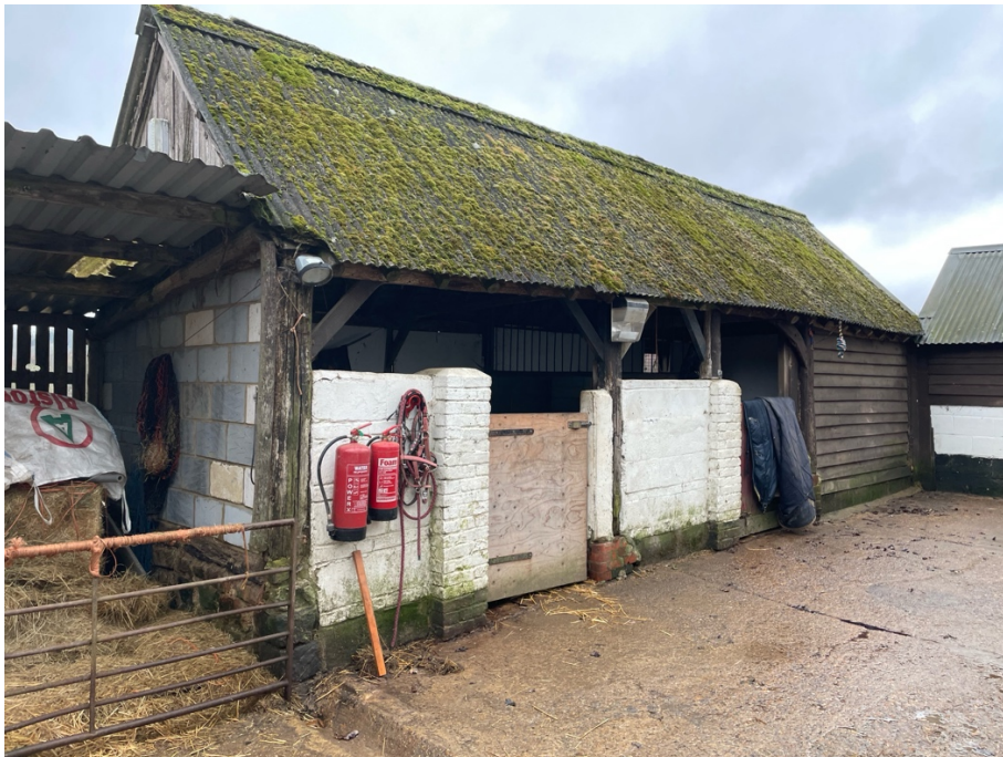
Photograph of the Southern Building
