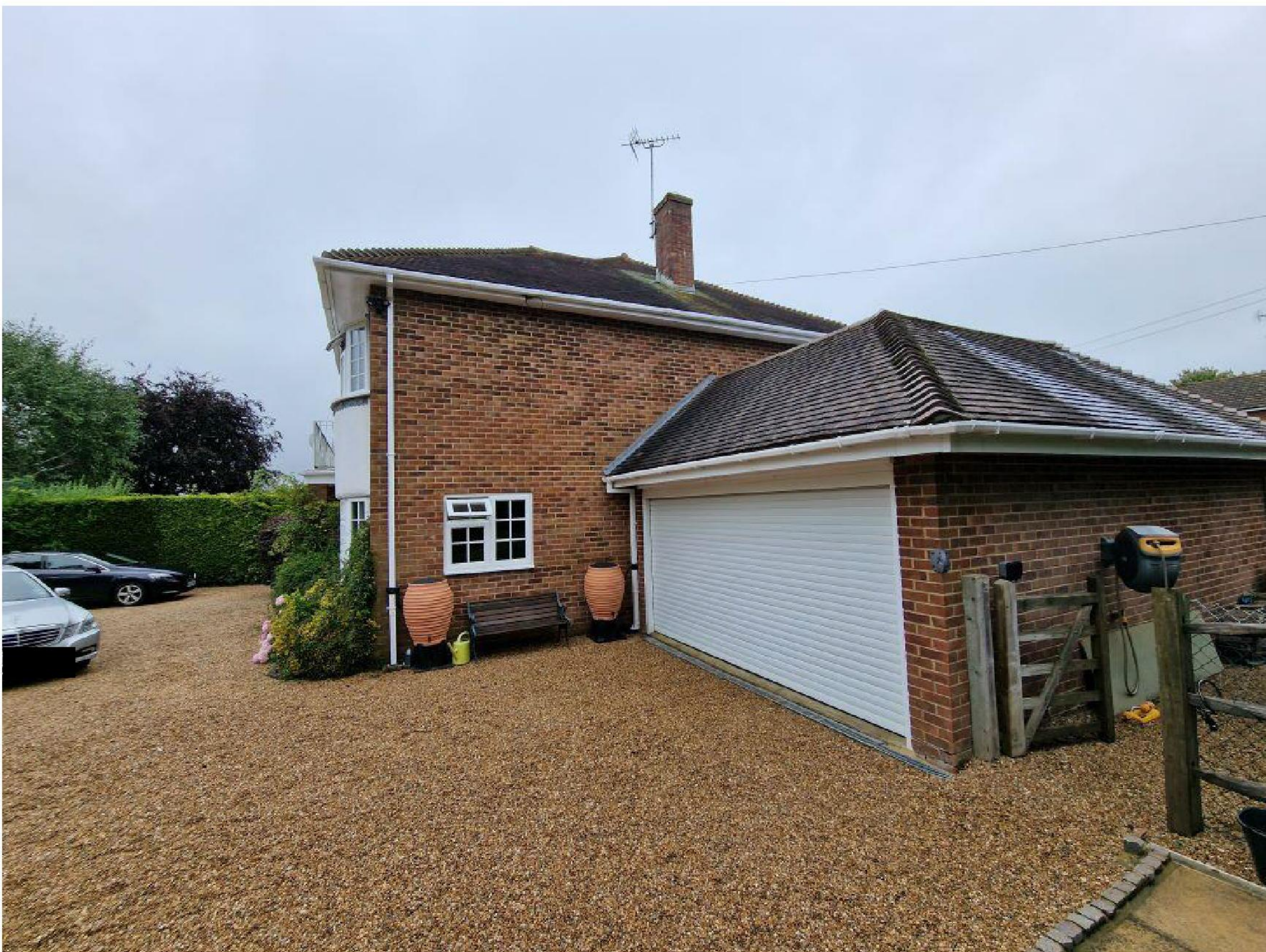
Existing Garage from the south west
