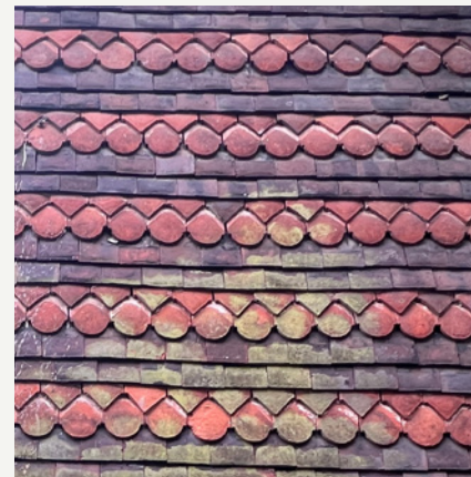
Clay Hung Tiles to North East Wing Courtyard
