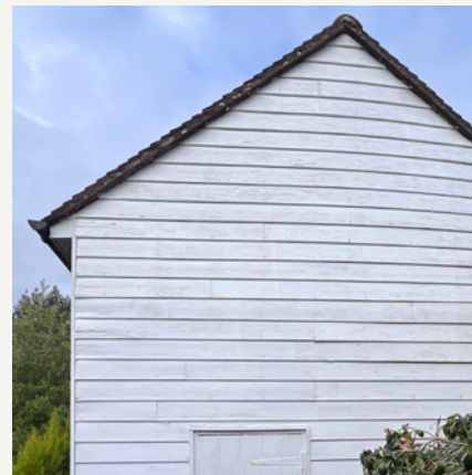
Outbuildings: white painted timber boarding
