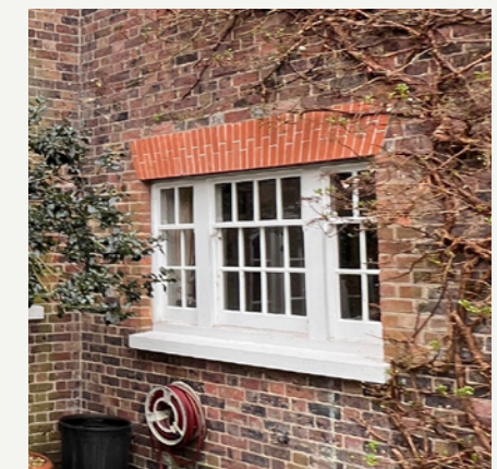
Modern openings and brickwork / lintels
