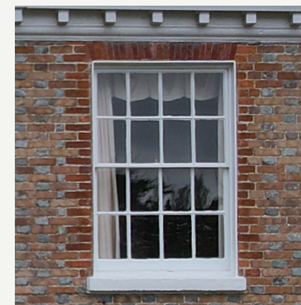
Diaper pattern red brick and grey headers. Deep wooden modillion eaves cornice. Modern White Painted Timber Sashes.
