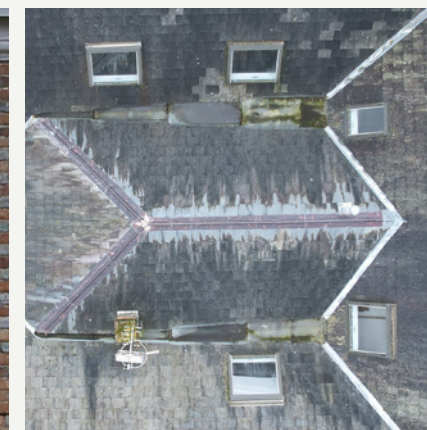
Steeply pitched replacement slate roof with 2 pedimented dormers.
