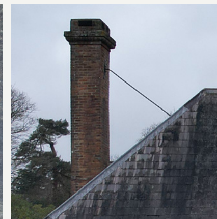
Brick chimneys with metal supports
