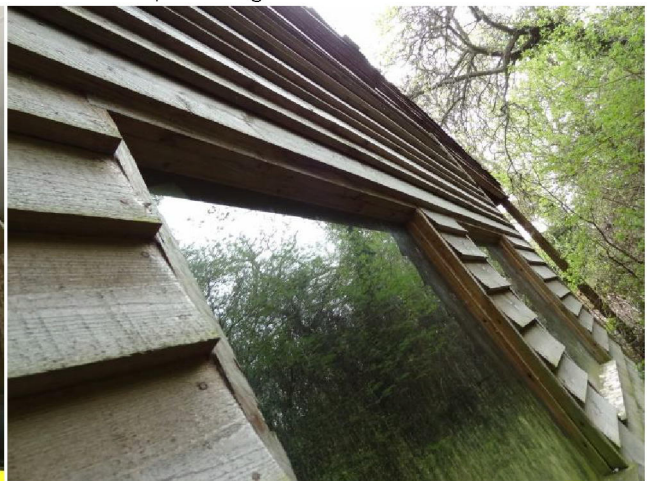
Windows and boarding tightly fitting to the west face
