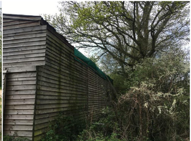
North face of the barn, sound construction
