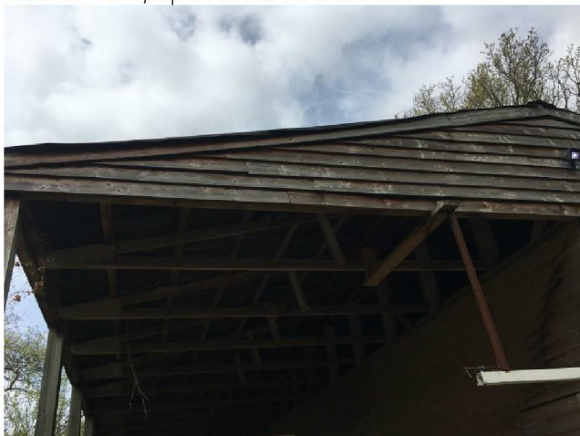
Exposed south face of roof void
