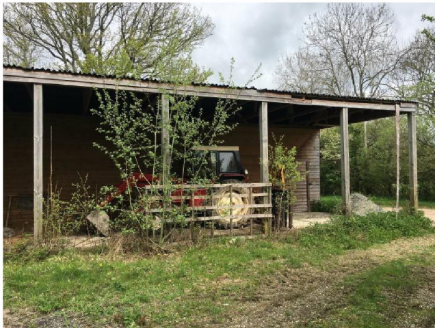
Exterior view, open sided to the south
