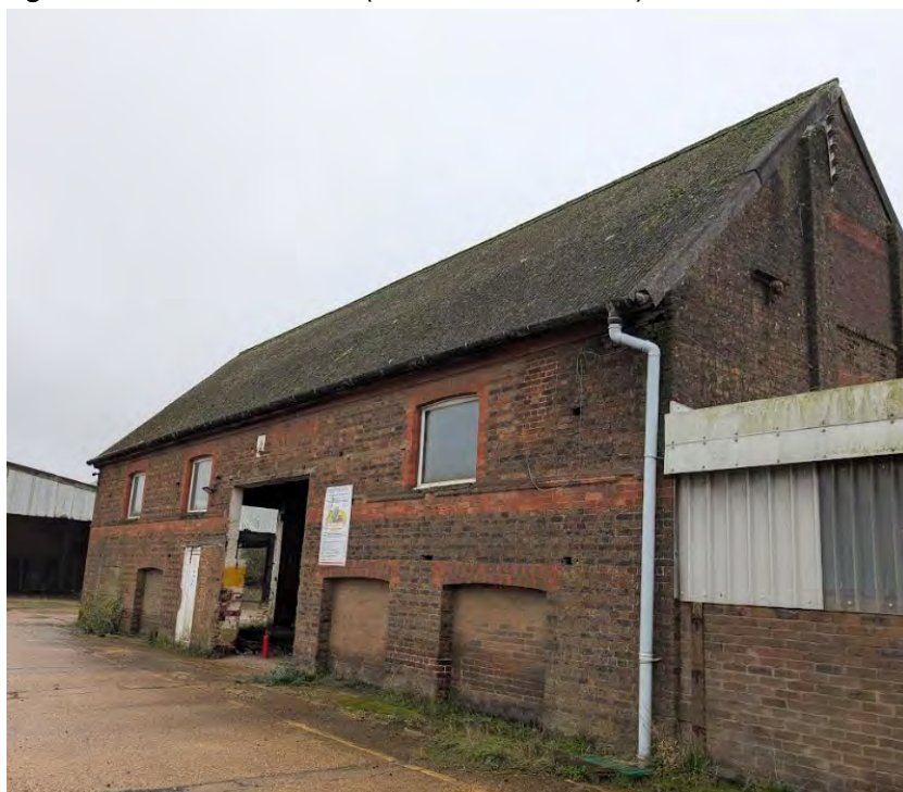
Figure 10. View of B4a on site (taken November 2024).
