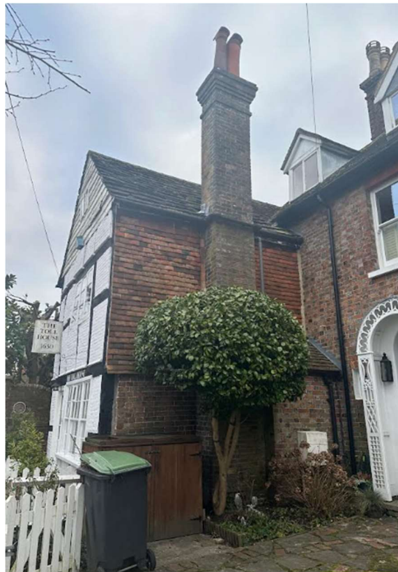
Figure 3 – Image of Chimney
