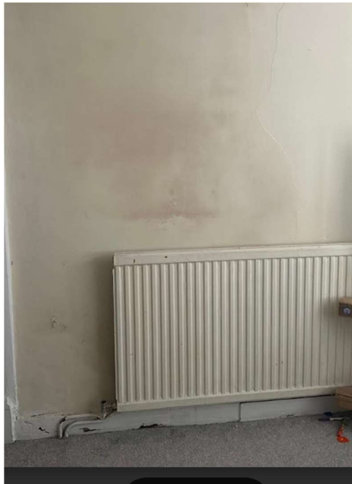
Figure 2 – Image of Bricked-up Fireplace
