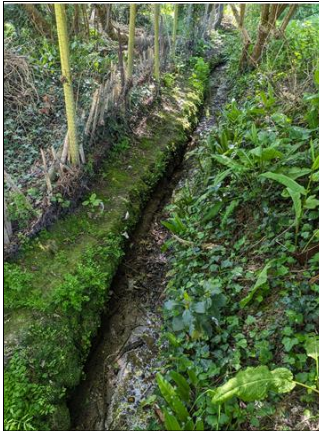
Figure 4-2 Ordinary watercourse observed on the site walkover
