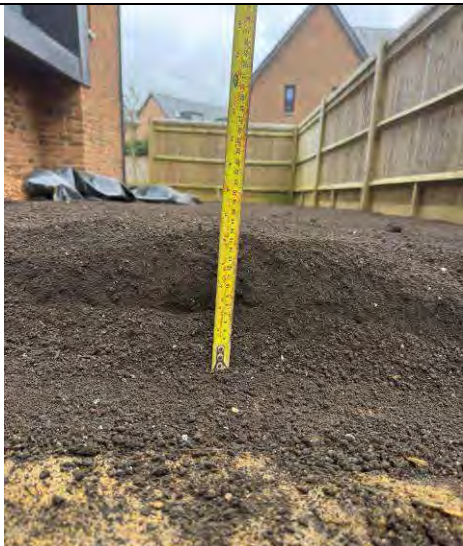
Plate 3: As plate 1, depth of topsoil provided approximately 0.15-0.16m.
