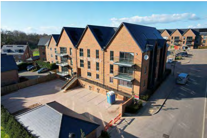
Plate 14: Looking towards the site from its north east side, looking north west.
