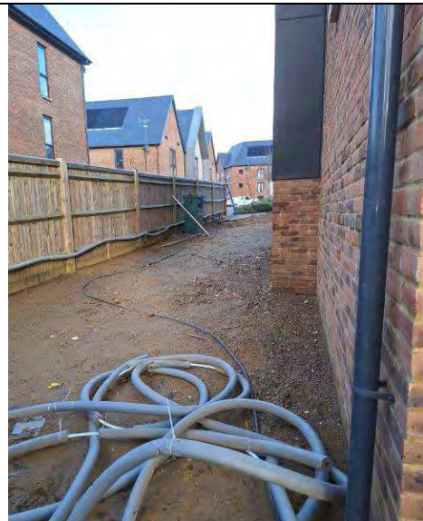
Plate 34: Side area to the west of the apartment, presumed to be soft landscaping.
