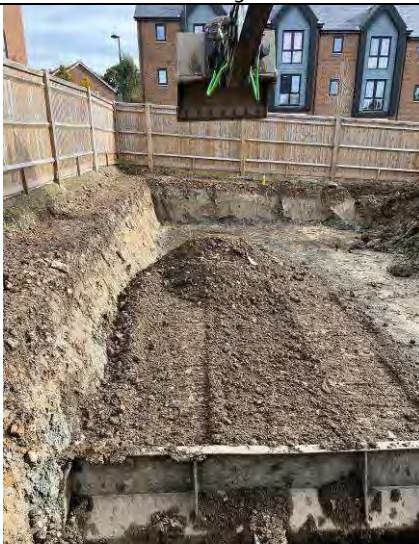
Plate 3: Soils encountered as part of the groundworks on site. We understand some soils were removed that had been placed as part of the former Car Park/Compound area. Replacement soils within the proposed soft landscaped areas.
