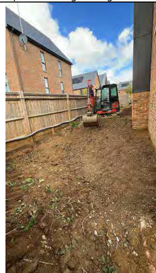
Plate 4: Placement of the subsoil in the western side of the site. We understand that this is the works to install some of the growing medium.
