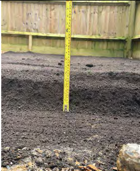
Plate 1: Topsoil placed in garden areas, depth of topsoil provided (approx. 0.13-0.14m).
