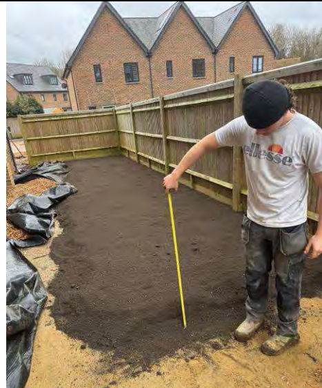
Plate 2: Looking southwards across the soft landscaping on the western side of the site. Topsoil placed over sandy subsoil visible at depth.
