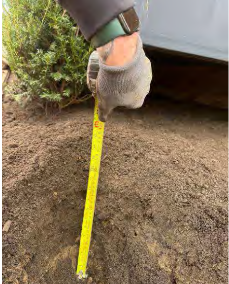
Plate 27: Topsoil placed in the soft landscaped planted area to the north east of the site, approximately 300mm cover material.
