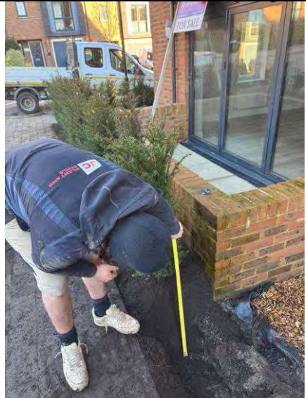
Plate 21: Additional topsoil added to the front (northern end of the site) soft landscaped area, looking west. Soils placed, photographic evidence of soils in the planted area.
