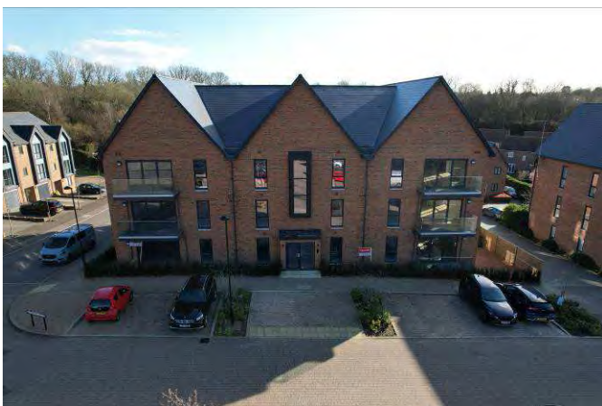
Plate 5: Looking southwards towards the northern end of the site. The planted up soft landscaping visible around the perimeter of the site.
