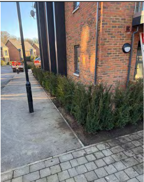
Plate 26: Completed planting and topsoil placement along the eastern side of the site, looking southwards.
