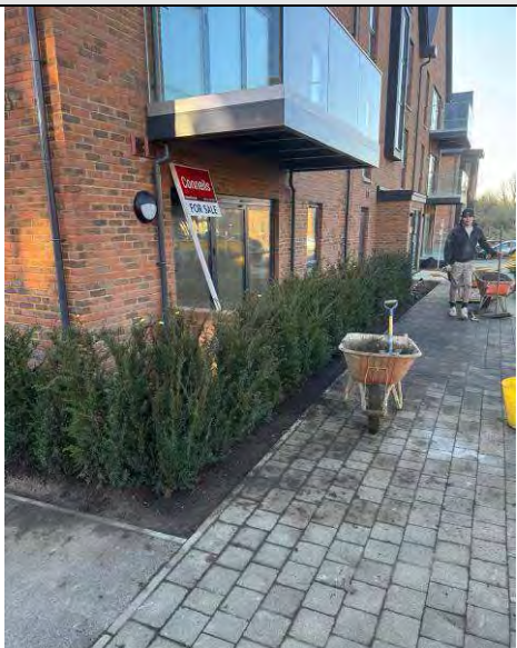
Plate 25: Completed planting and topsoil placement along the northern side of the site, looking westwards.
