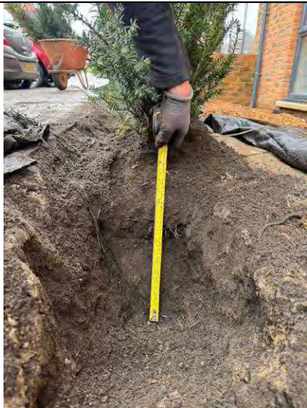
Plate 29: As plates 27 & 28, topsoil placed in planted areas to the north of the site.
