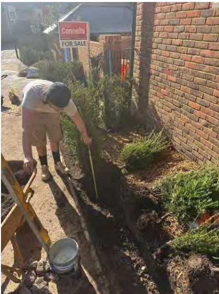
Plate 17: Topsoil provided in the planted areas. Region of soft landscaping areas to the east of the site, Kilnwood Avenue (east).
