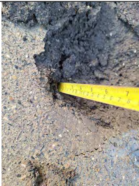
Plate 8: As plates 6 & 7, depth of topsoil placed.
