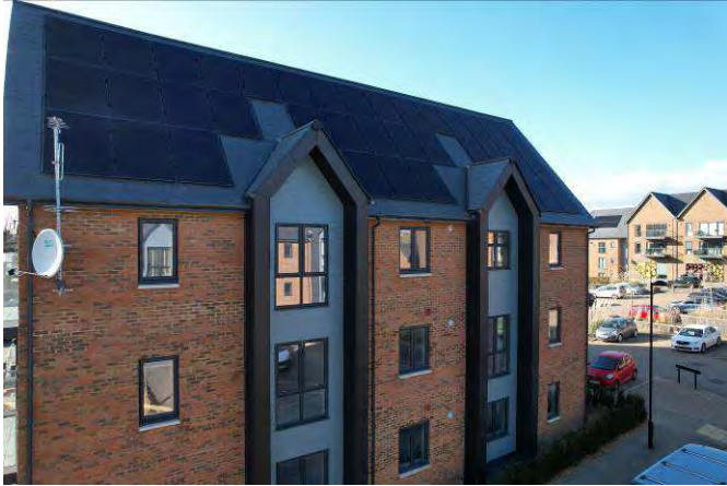
Plate 1: The site looking north west.
