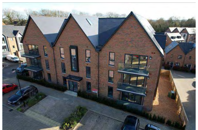
Plate 6: The northern and western side of the site looking southwards. The soft landscaped area at the perimeter is shown planted. The region to the west is currently not planted.
