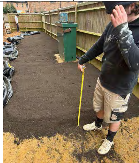
Plate 4: Placed topsoil along the western soft landscaped area. Sandy subsoil visible at depth.
