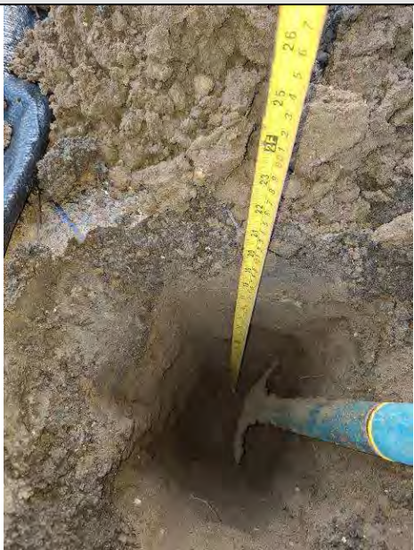
Plate 13: Spot Pit 3, depth of subsoil provided.
