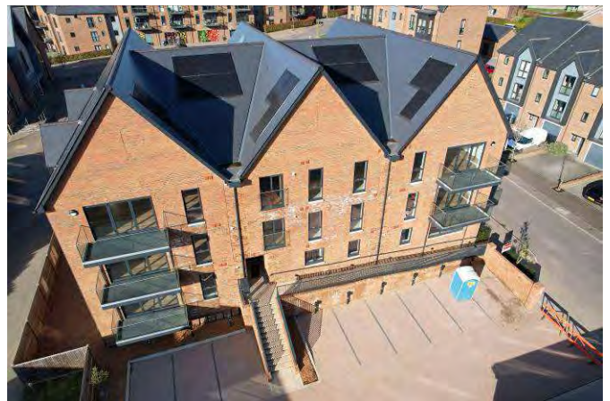
Plate 12: Looking northwards across the rear of the site (southern end of the site), looking towards the apartment block. Soft landscaped areas surround the car park at its southern, western and north western end.
