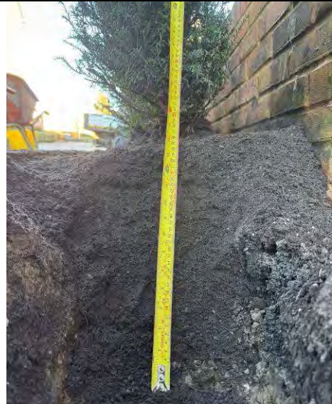
Plate 22: As plate 21, topsoil placed in the soft landscaped planted area to the northern end of the site, approximately 300mm cover material.
