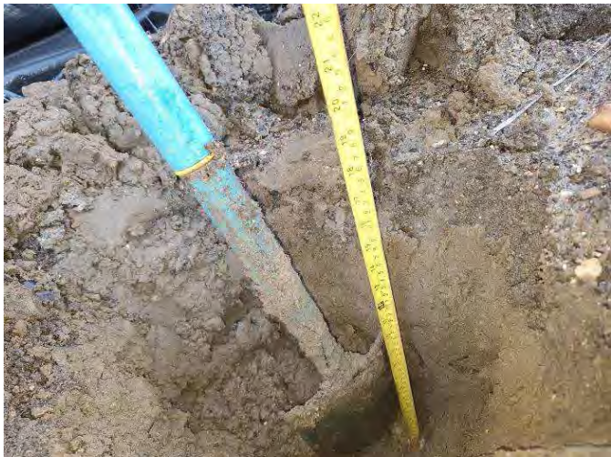
Plate 2: Spot Pit 1, depth of subsoil 0.45m.
