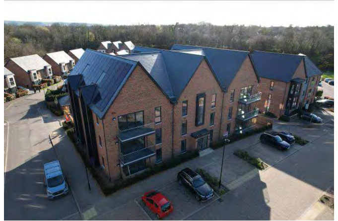
Plate 2: The northern end of the site showing the soft landscaping to the front of the apartment block.
