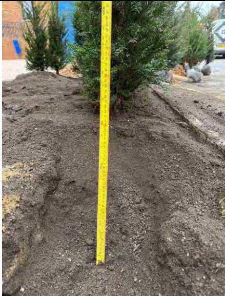
Plate 11: Additional topsoil added to the rear (south eastern end of the site) soft landscaped area, looking north. Soils placed, photographic evidence of soils in the planted area.
