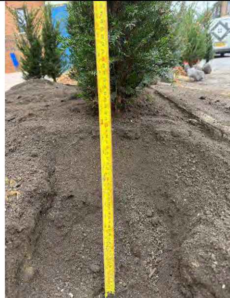
Plate 12: As plate 11, approximately 0.2m-0.3m of topsoil to the planted area at the front.
