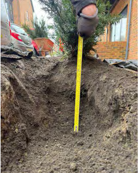
Plate 28: As plate 27, topsoil placed in planted areas to the north of the site.
