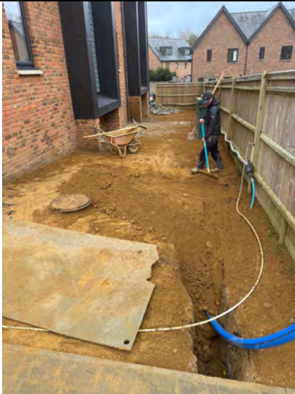
Plate 1: Soft landscaping along the western side, we understand that this is the works to install the services within the existing soils.
