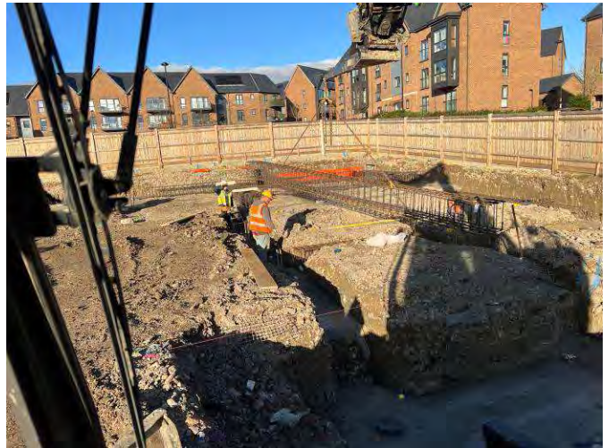
Plate 2: Work underway to install the footings within the soils placed as part of the initial formation level soils and lower layers of the growing medium.
