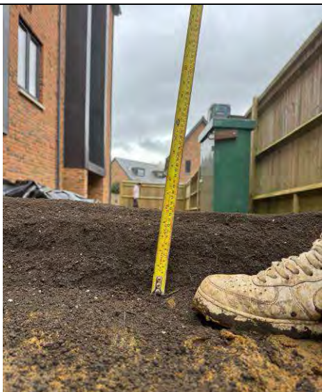
Plate 5: As plates 1 & 3, depth of topsoil provided approximately 0.15m.
