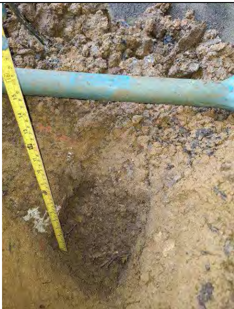
Plate 29: Spot Pit 7, soils encountered. Rootlets noted encroaching into the pit.
