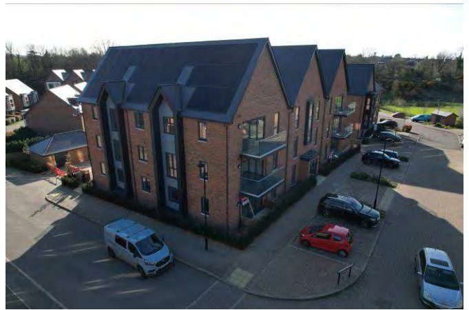
Plate 4: As plate 3, looking south west towards the apartment block from the northern end.
