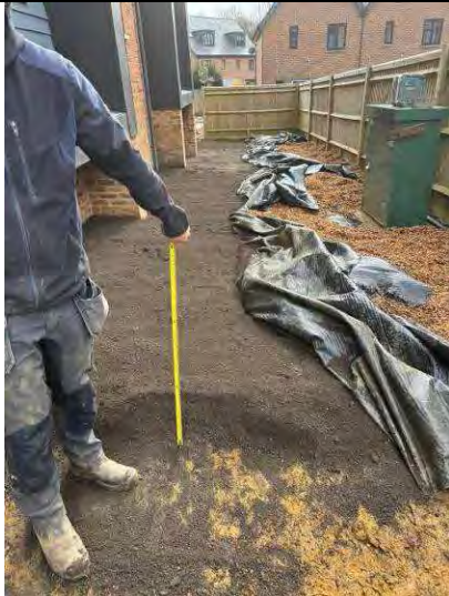
Plate 9: Additional topsoil added to region to the north, as topsoil placement is continuing up the soft landscaped area.
