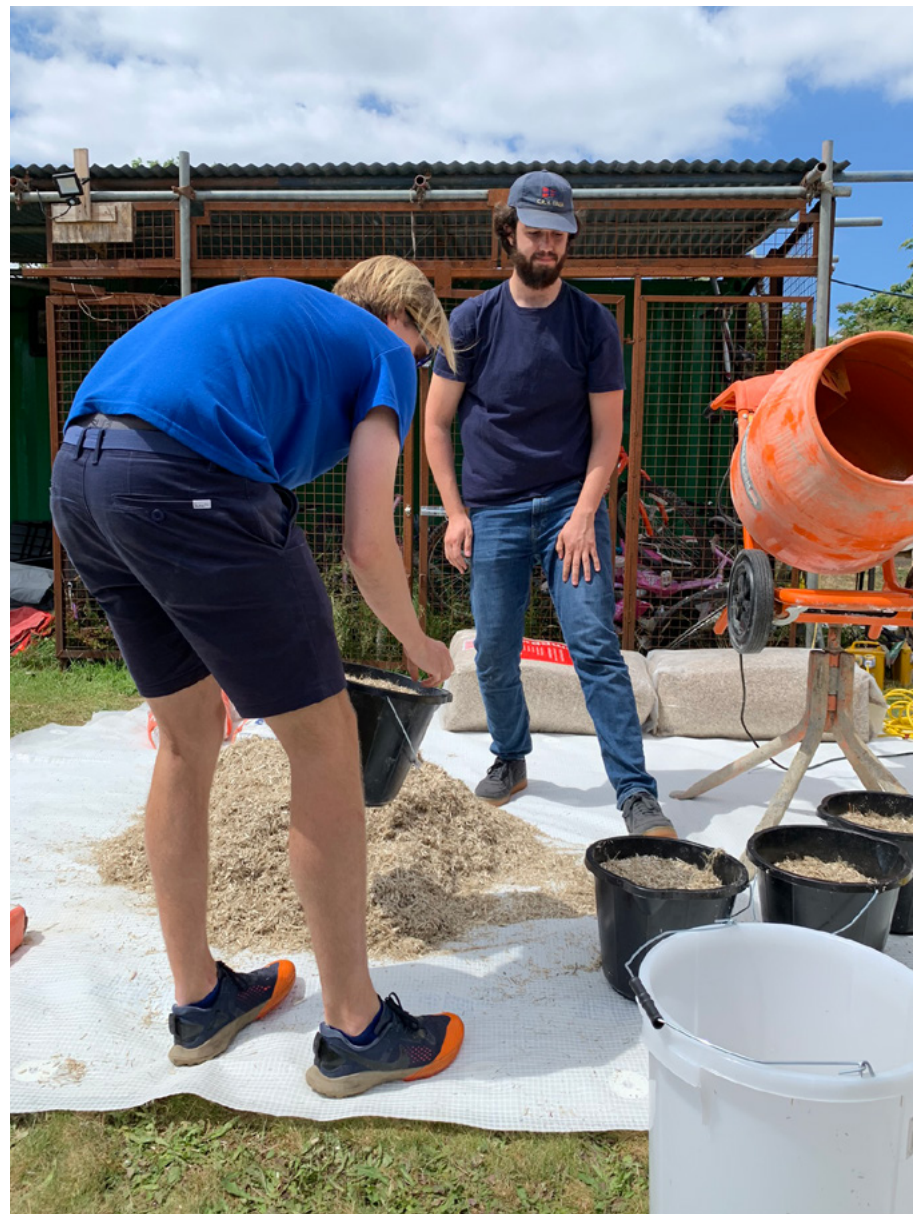
Photograph taken by Benjamin Machin during hempcrete building workshop
