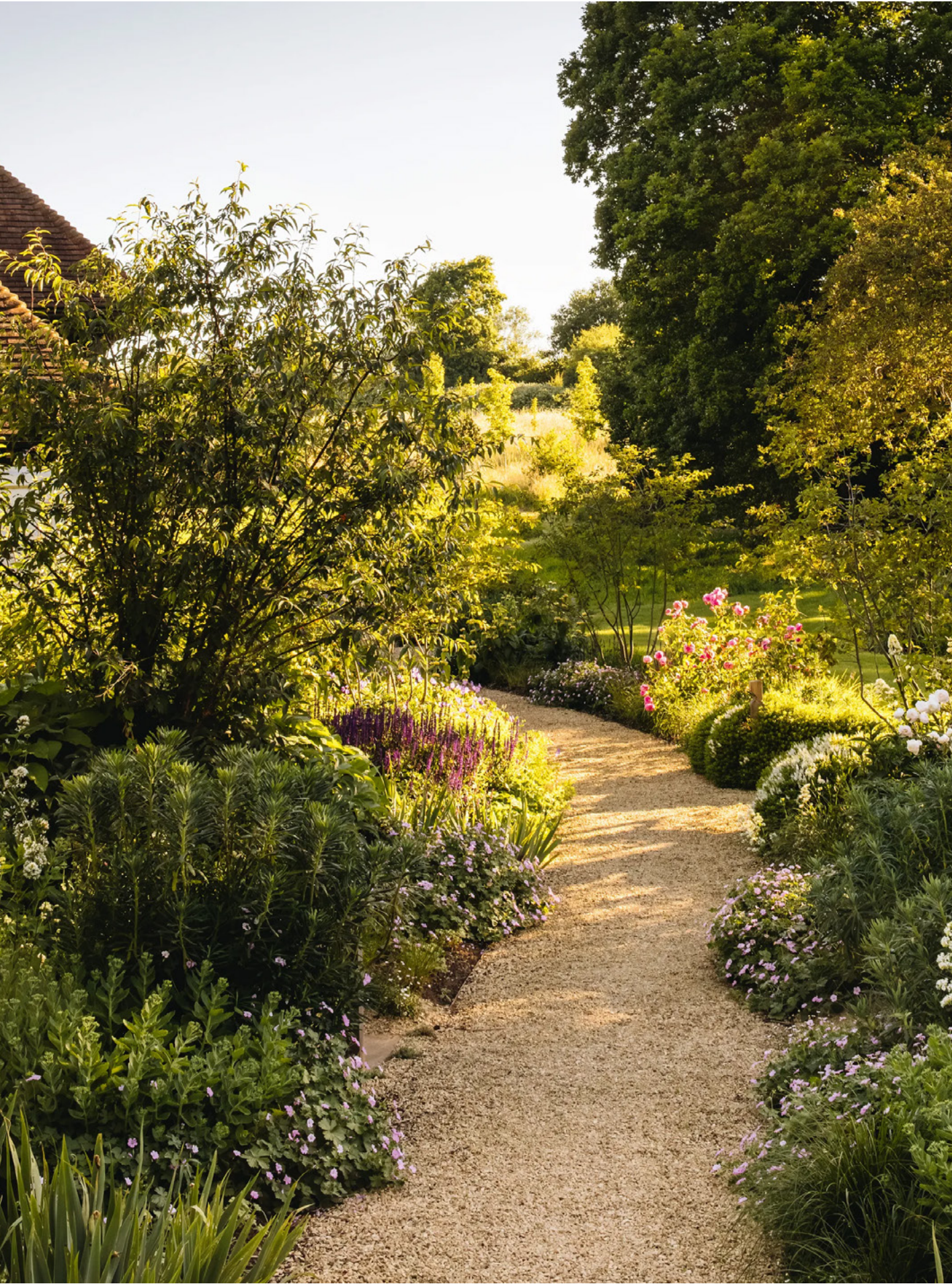
Cottage garden in Kent denoting permeable resin-bound gravel pathways for accessibility and to resolve level changes for wheelchair users
