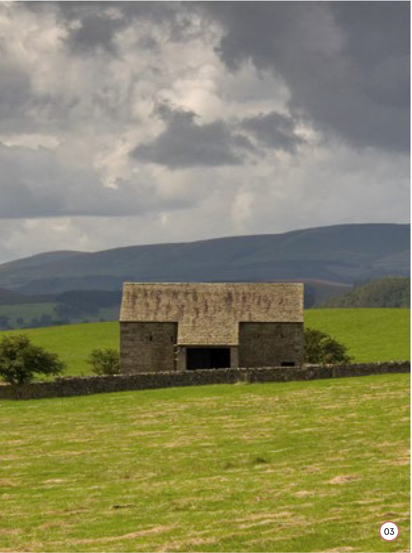
Extended catslide roof form
