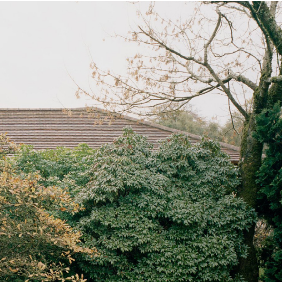
Reference of a pitched roof set within a rural landscape
