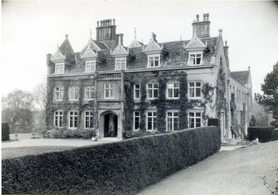
Figure 4.25: Photograph 1883 East Entrance front of the house 53
