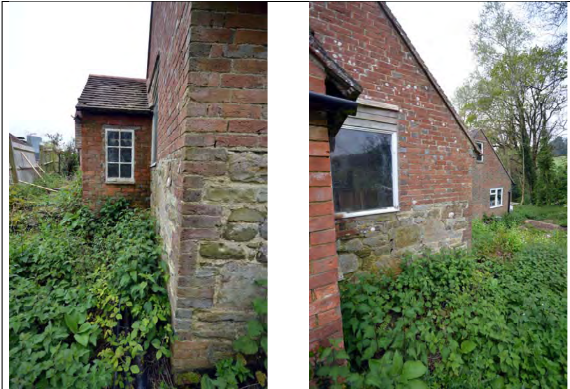
Plate 4: The masonry base at its northeast corner and east side
