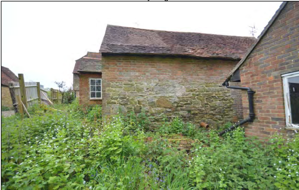
Plate 3: The north side of the north ancillary range, earlier masonry, later brick above
