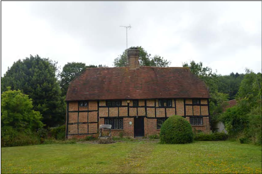
Plate 1: The south side of the house as arrived at by the 18 th century showing the contrast in construction between the rebuilt western end and its predecessors to the east
