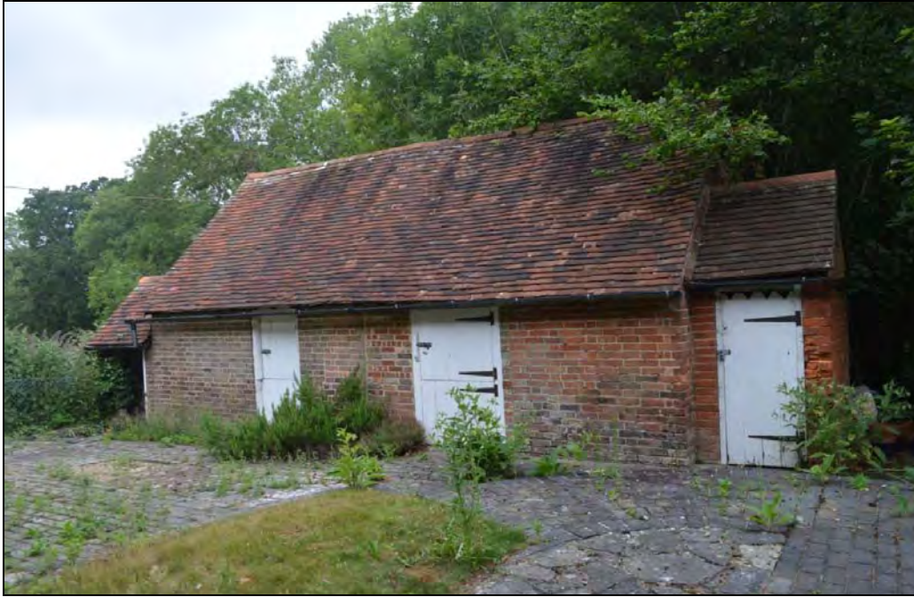
Plate 2: The south side of the north ancillary range
