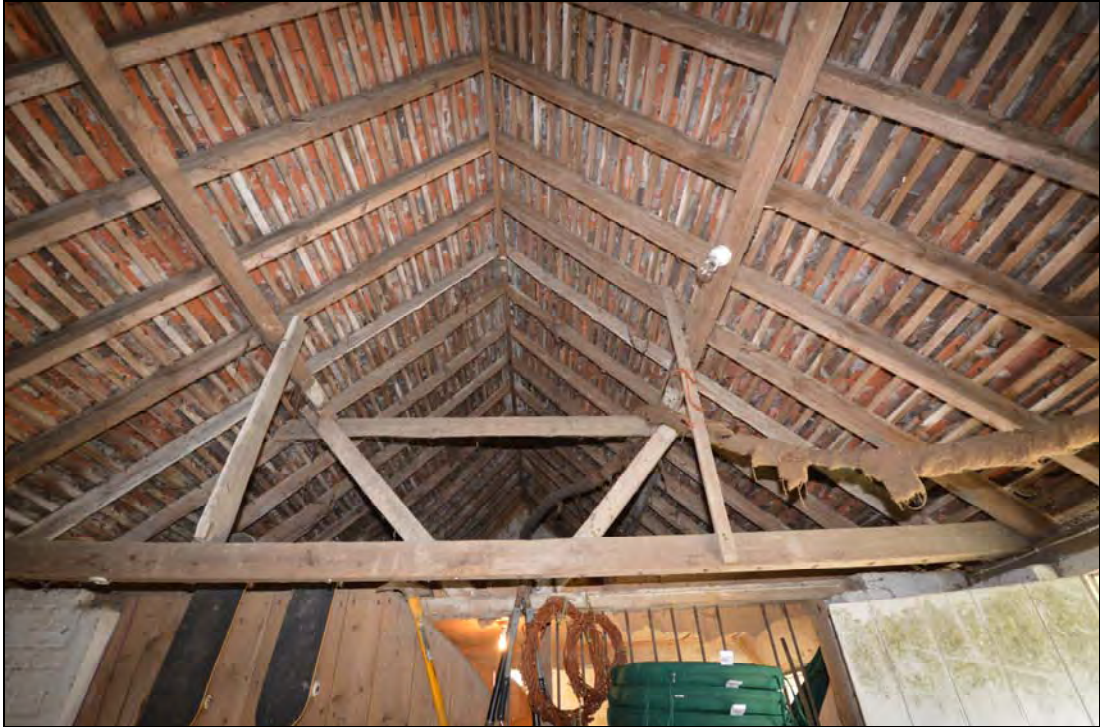
Plate 7: The consistent roof over the various parts of the main range looking east
