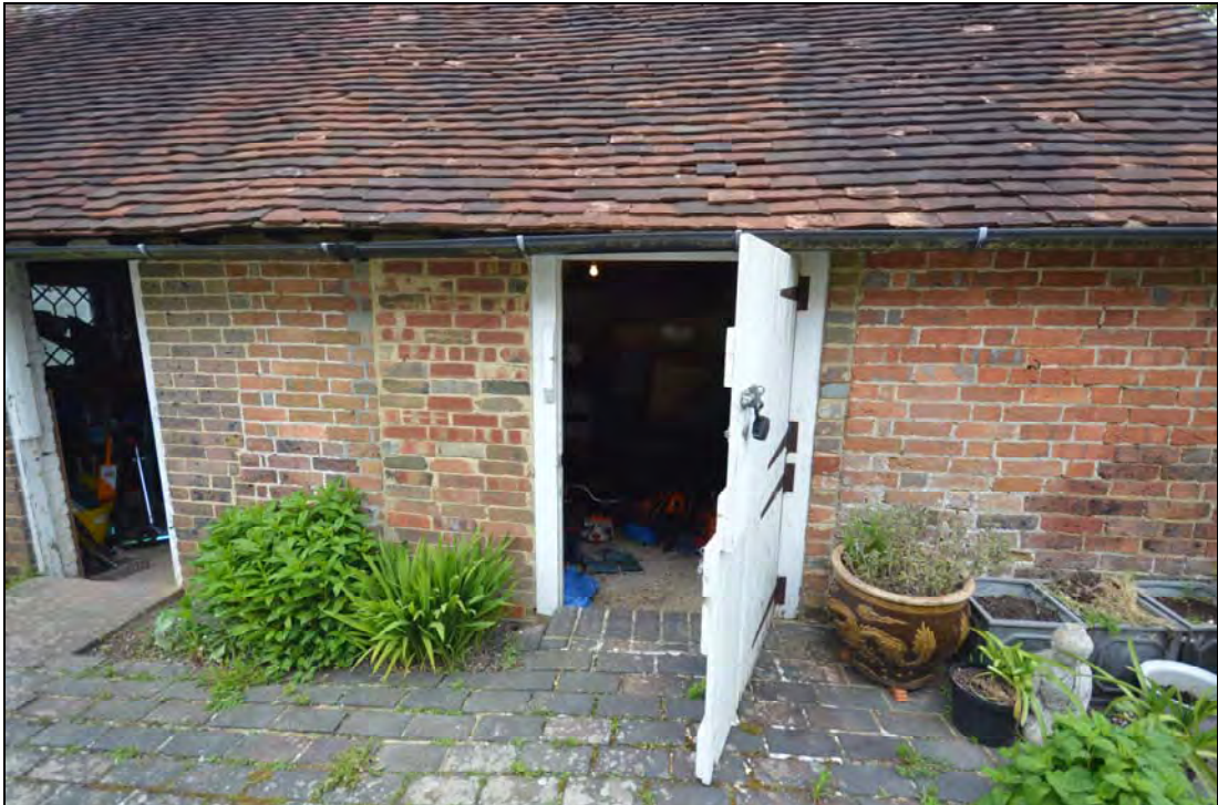
Plate 5: The south front showing Sussex bond brickwork to the east side of the current entrance
