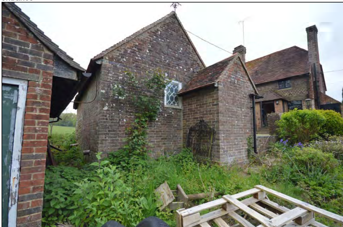
Plate 6: The new west end of the range in Sussex bond with integral single-light window
