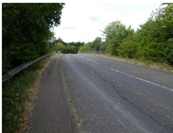
Photograph taken 21/07/2026, of the derestricted A23 slip road approaching the flyover just before the site entrance. It show some of the differences in road heights which have an effect on vehicle visibility
