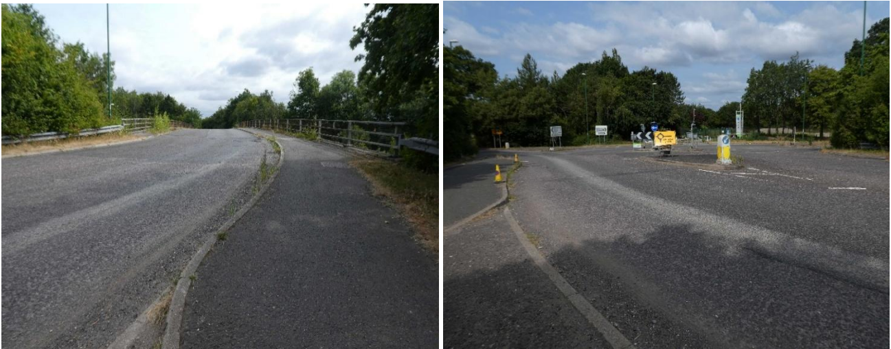
Photographs taken from the site entrance 21/07/2026. Left the view of the roadway to the east and the slip road flyover. Right the view of the roadway to the west including the roundabout.
