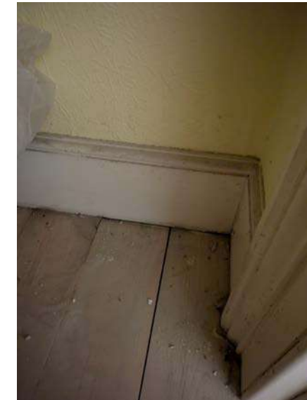
Original skirting to S18
