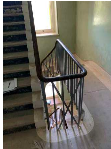
Example of existing stairwell balustrade retained
