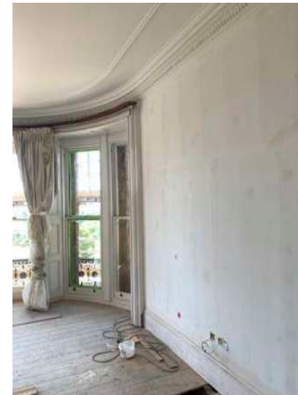
Example of cornicing and skirting retained
