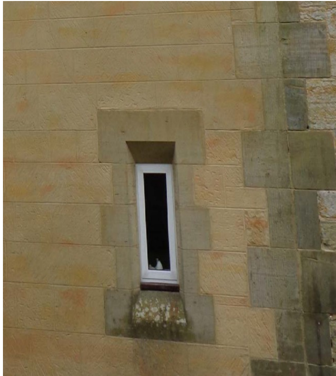
Left: Walls to match the existing rendered finish
