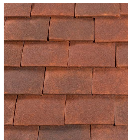
Right: Handmade plain clay tiles to the pitched roof
