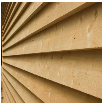
Left: Natural oiled timber cladding, fixed horizontally
