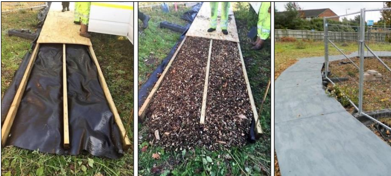
Image 6: Showing an example of a ply boarding above woodchip system of temporary ground protection.
