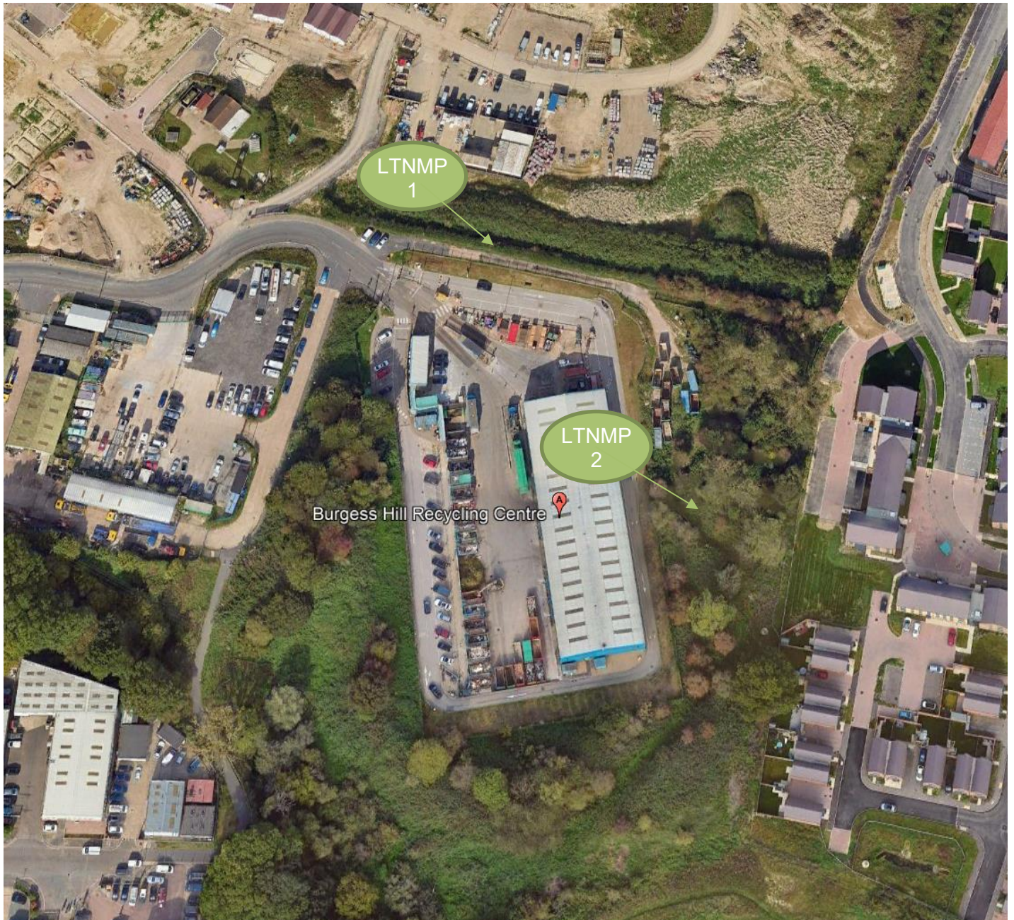
Figure B: Location Aerial View and Identification of LTNMP 1 & 2,
