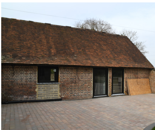
Fig 7, South Elevation of Cart Sheds
