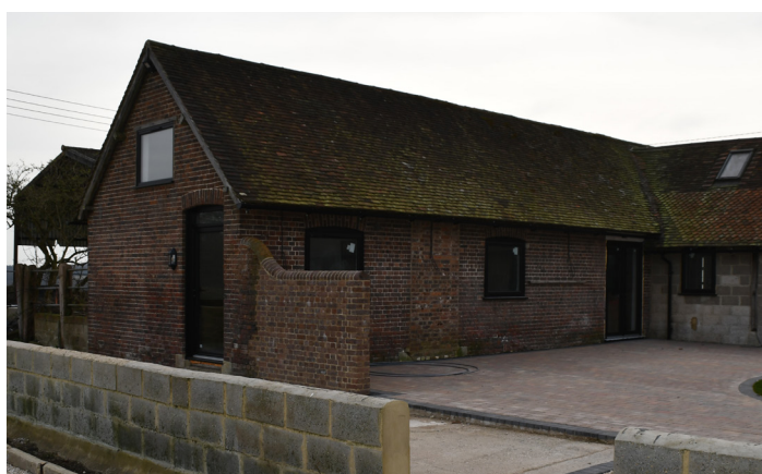
Fig 3, The Stable, North & East Elevations
