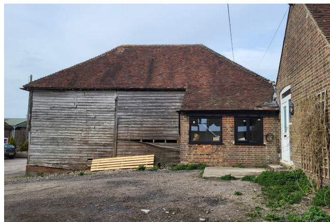
Fig 10, The Barn, South Elevation
