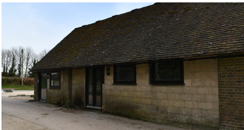
Fig 8, North Elevation of Cart Sheds
